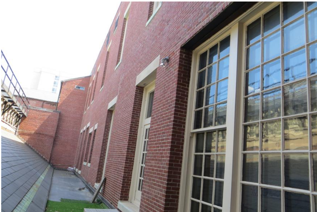
Figure #11. East elevation second story and attic level windows (from first story roof, looking south). July 2016.
