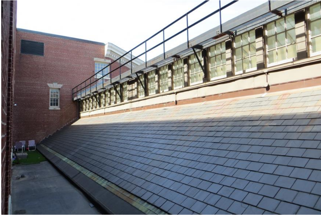
Figure #11. Monitor roof (from first story roof, looking north). July 2016.
