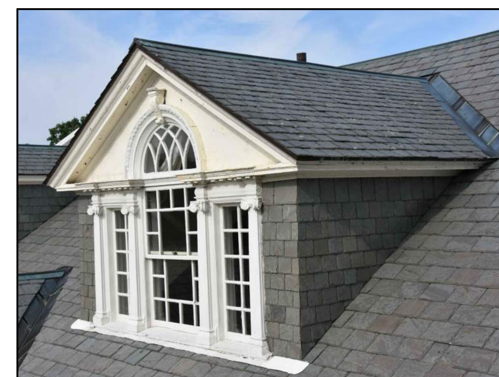
6 ROOF DORMER - EAST
