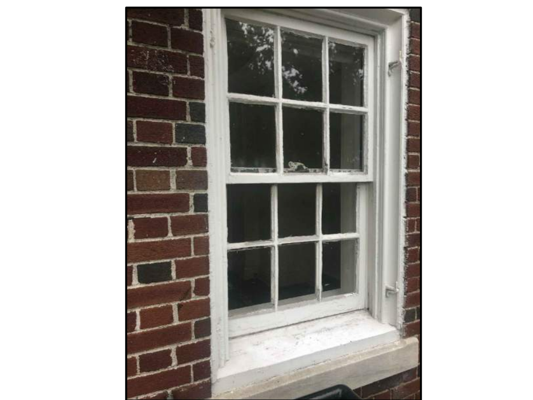
6 TYPICAL WINDOW CONDITION
