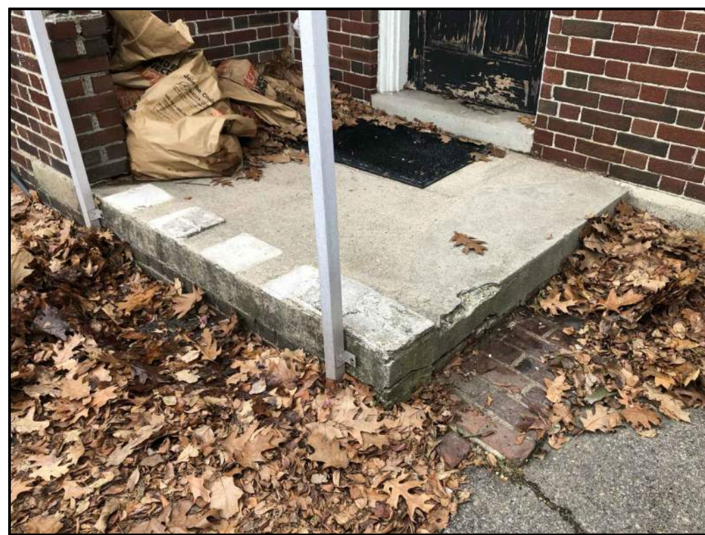
20 REMAINS OF EXISTING BALUSTRADE
