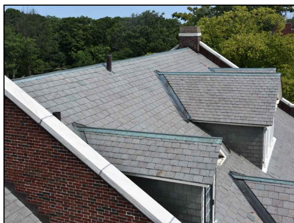
20 TYPICAL SLATE ROOF
