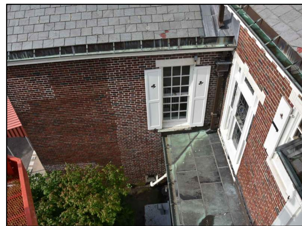
10 MASONRY JOINTS TO BE STAINED
