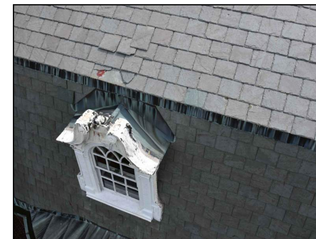
3 STEEP SLOPE SLATE ROOF
