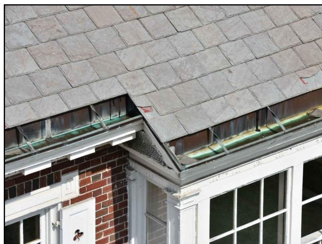
19 TYPICAL GUTTER CONDITION
