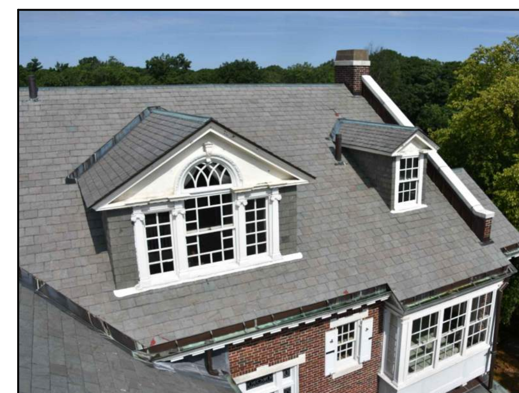
5 ROOF DORMERS - EAST
