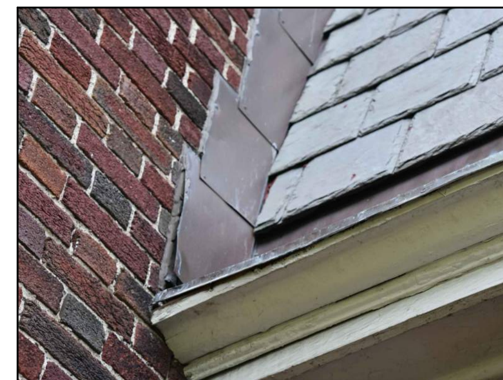
7 COPPER ROOF FLASHING
