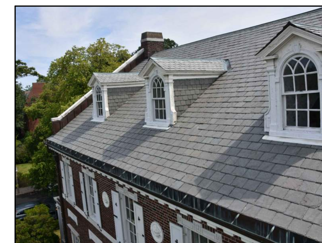
1 ROOF DORMERS - WEST
