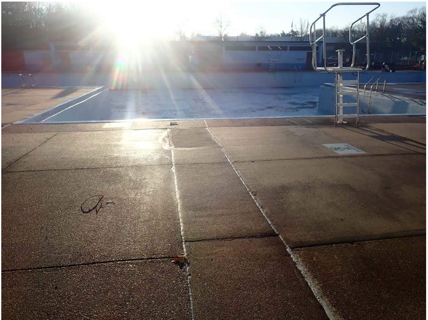
Photo 1 – View (from the North) of Olsen Pool located at 95 Turtle Pond Parkway in Boston (Hyde Park).
