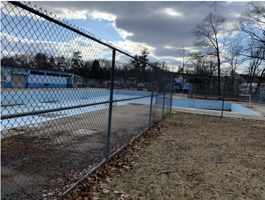
Photo 7 – View of Olsen Pool contained within the fence. The project area will not exceed the boundaries of the fence or deck footprint. As viewed from the northeast.
