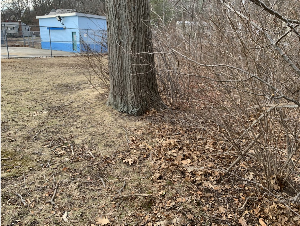
Photo 6 – View of the pool shed building to the north of the pool deck, as viewed from the east.
