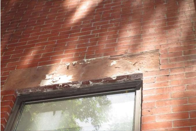
View of skimcoated and damaged lintels to be replaced with matching lintels
