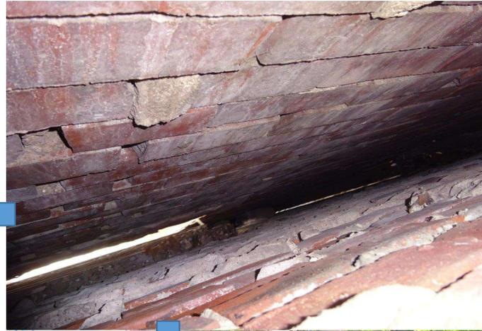
View of third-floor unit, cavity between inner and outer wythes due to water damage bowing out outer brickwork
