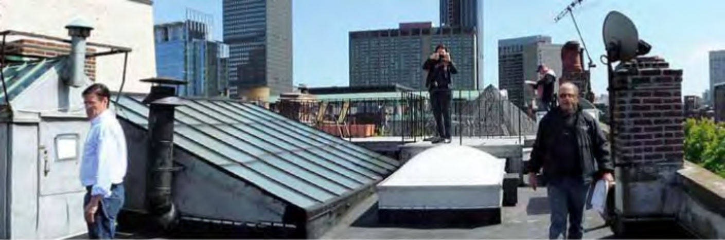
Existing Roof @ 315 Commonwealth Ave. looking South
