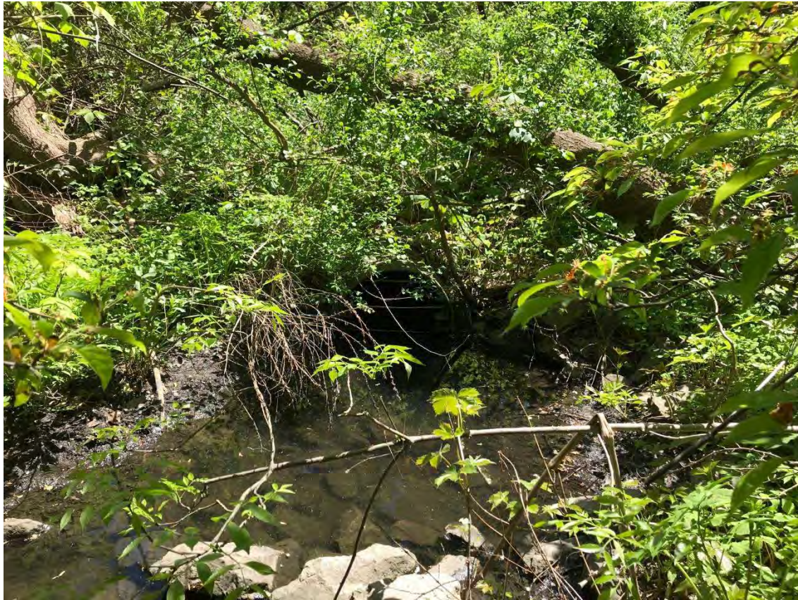
Photo 5: 18-inch diameter drain outfall (near WF 7-65)
