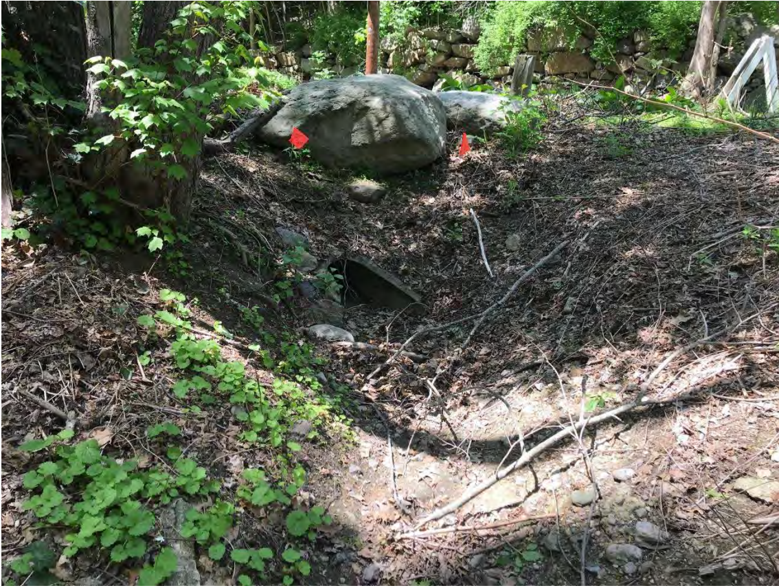
Photo 22: Stormwater drainage outfall at end of Hazelmere Road
