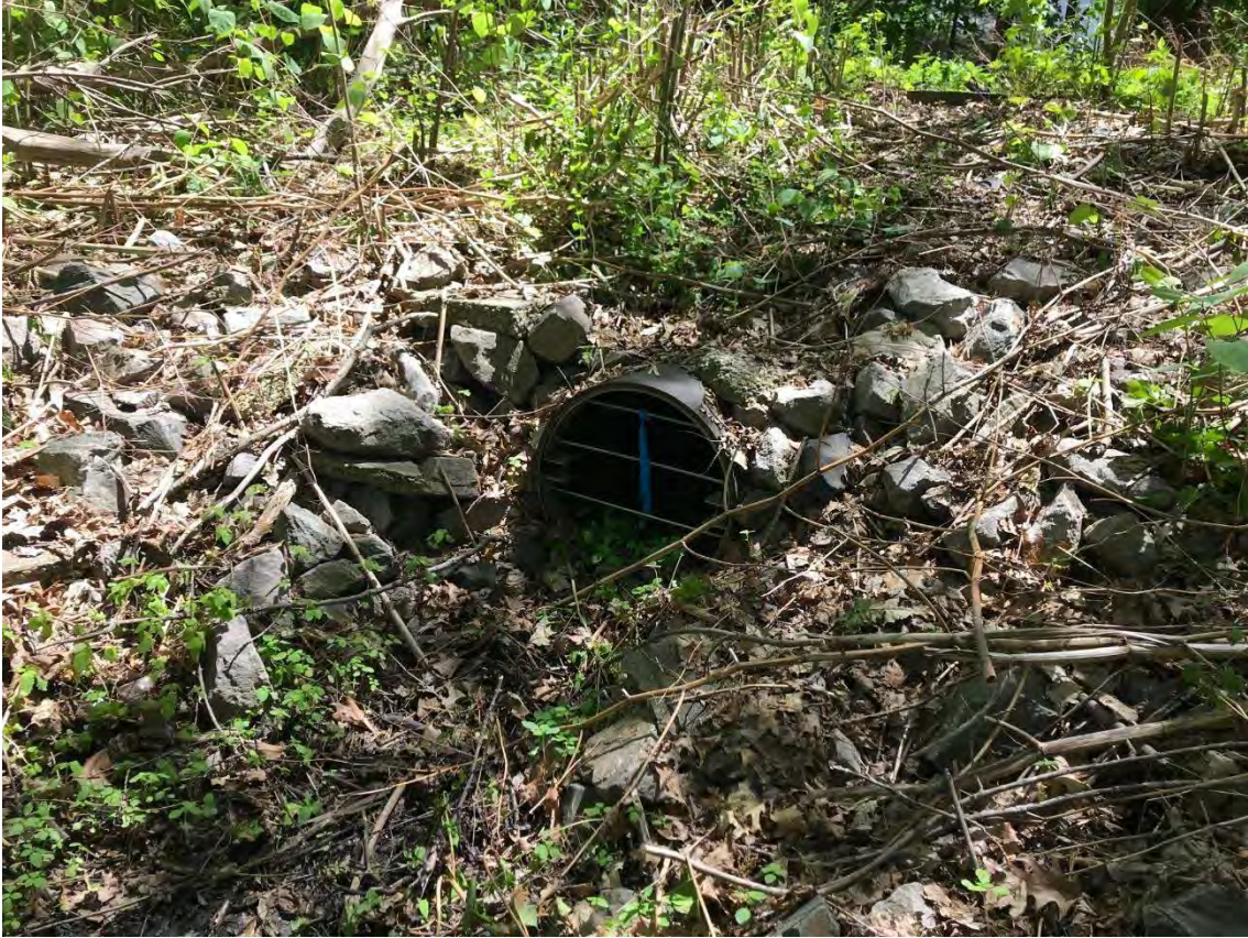
Photo 7: Drain outfall by WF 7-87
