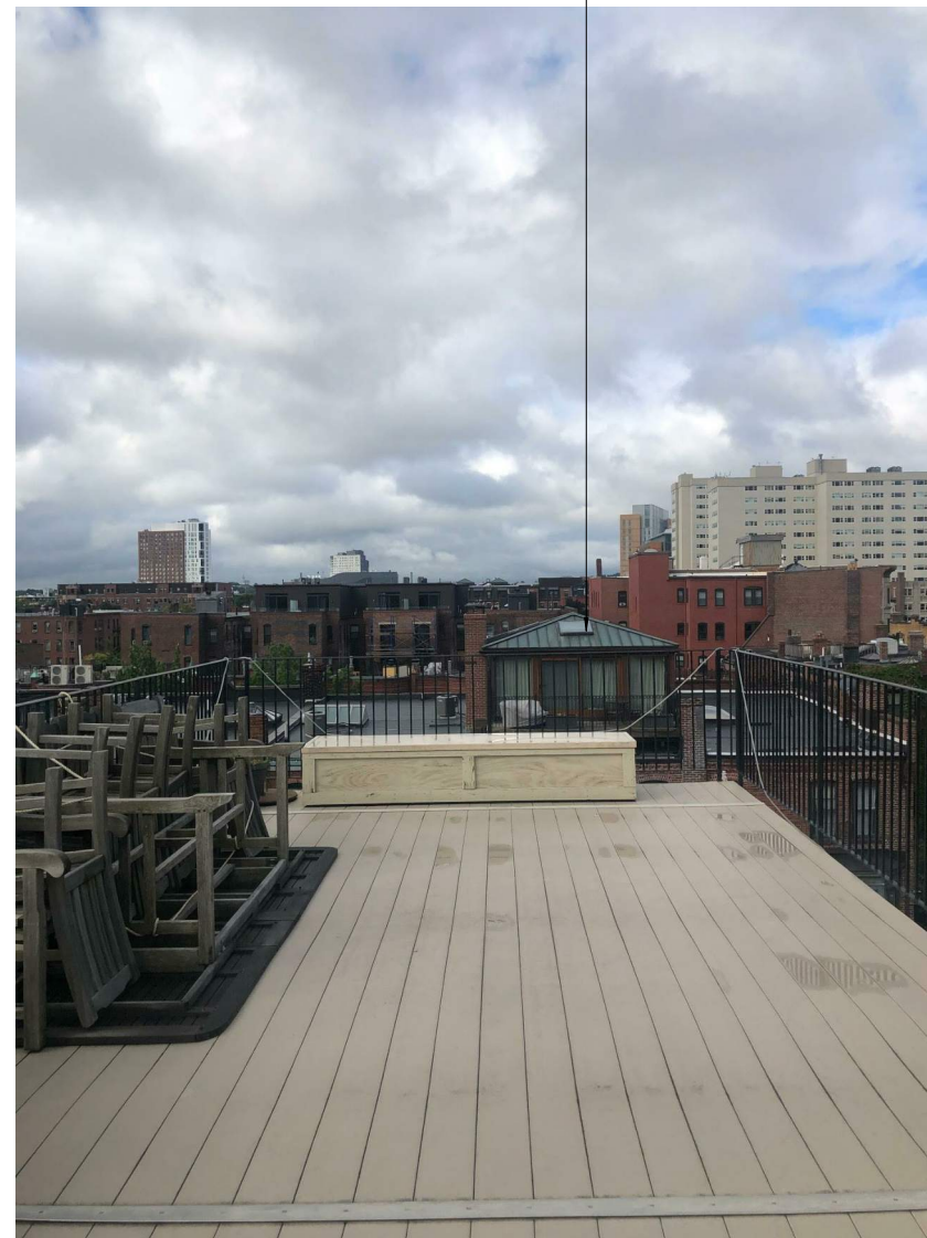
EXISTING ROOF DECK PHOTO 2
