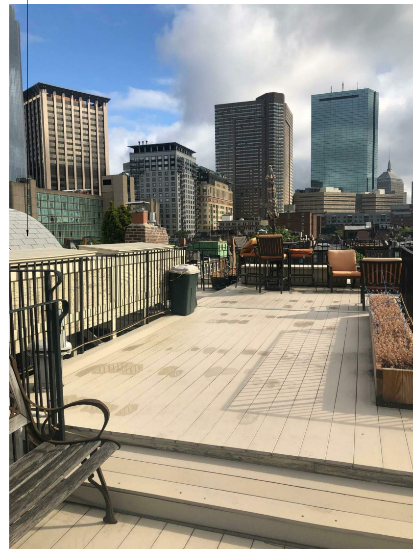
EXISTING ROOF DECK PHOTO 3
