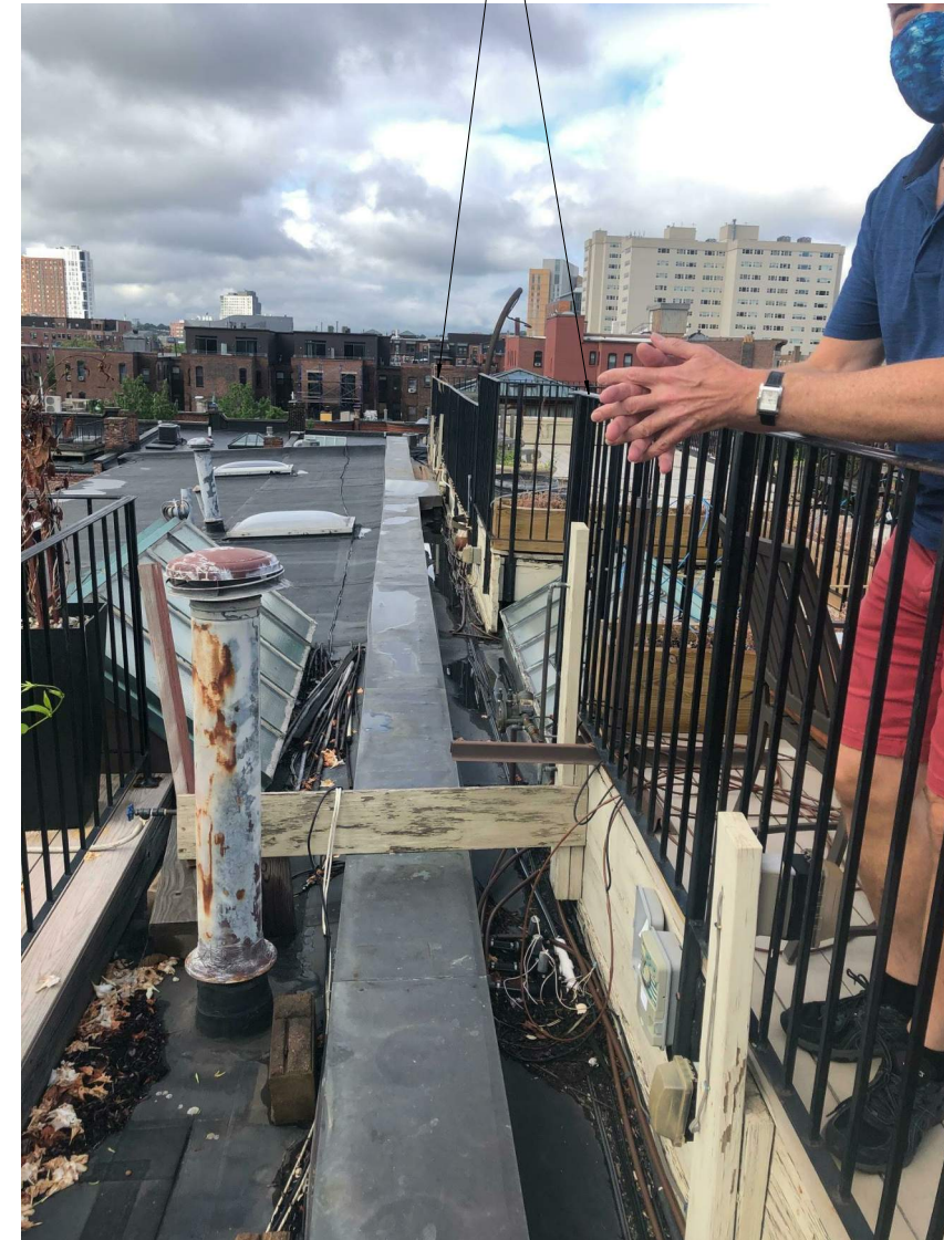
EXISTING ROOF DECK PHOTO 1
