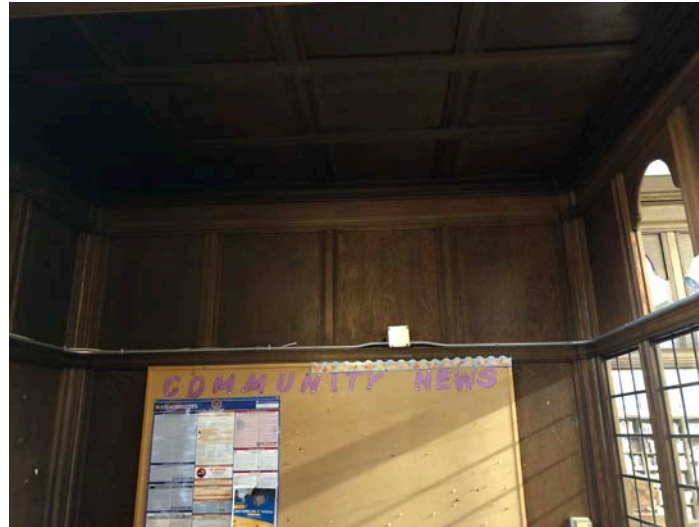
ENTRY VESTIBULE: Data wire will follow existing metal conduit
