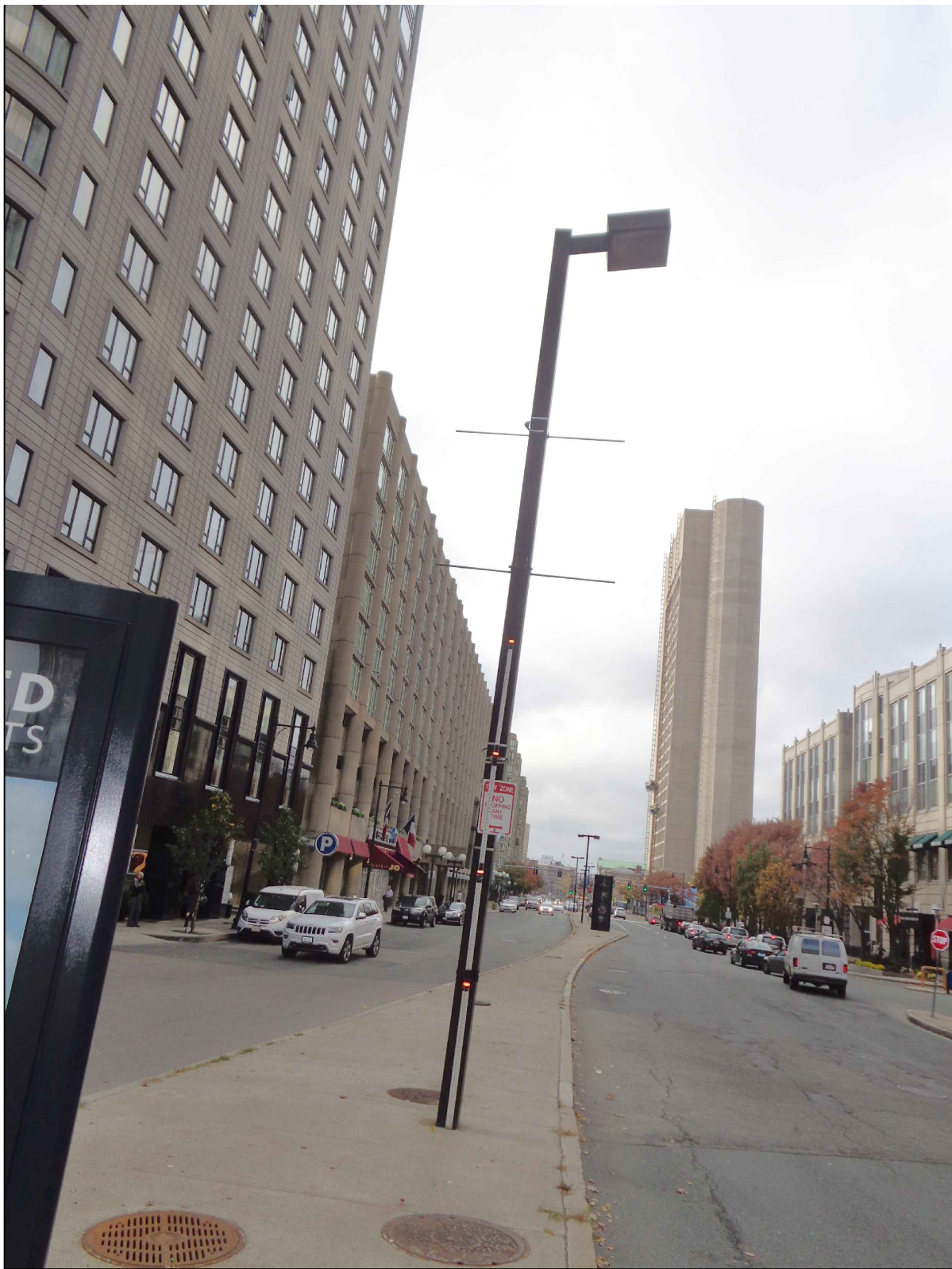
CONTEMPORARY SQUARE ALUMINIUM POLE EXISTING CONDITIONS - EXHIBIT X-17
