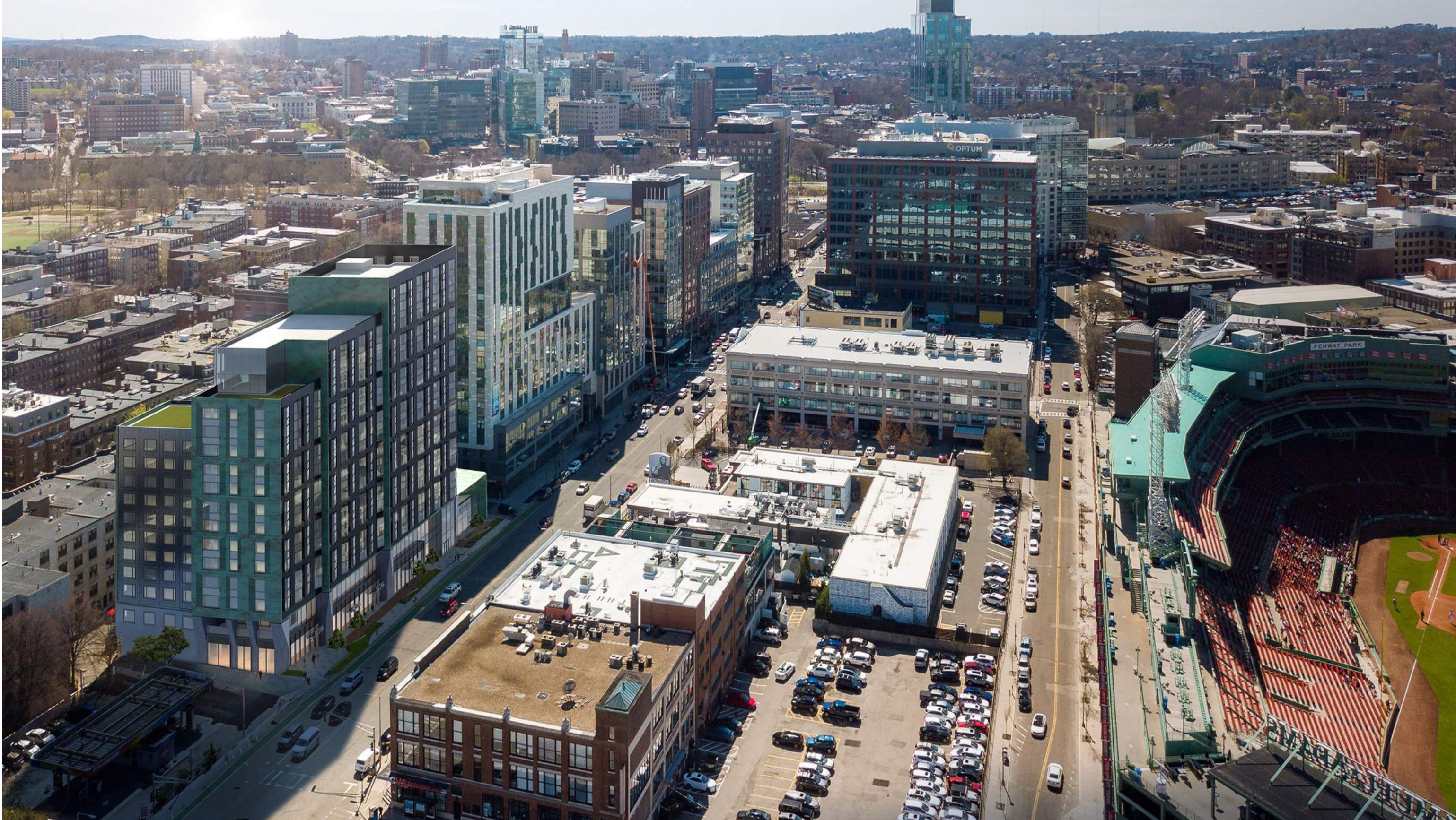
AERIAL VIEW | LOOKING WEST.
