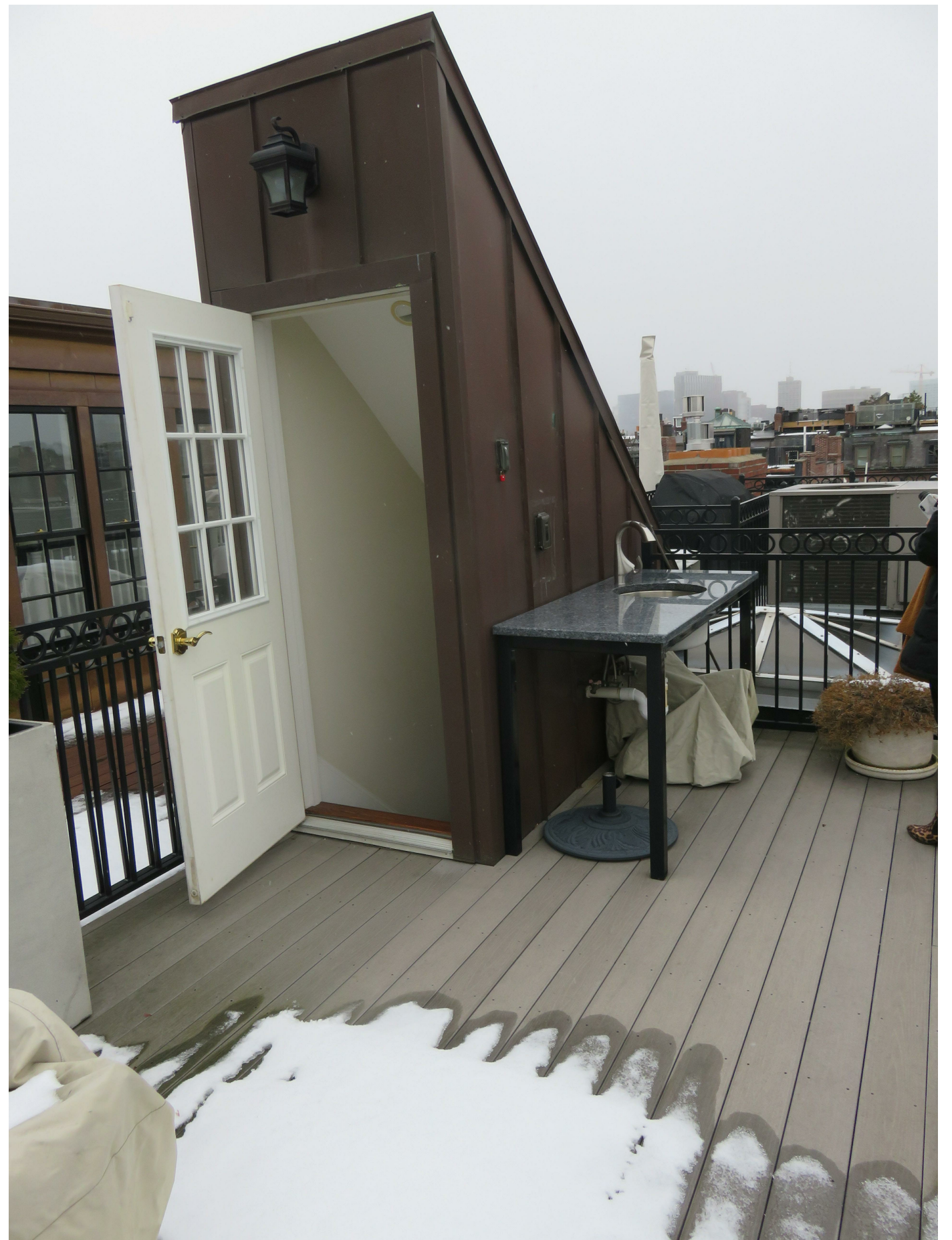
EXISTING ROOF DECK - HEADHOUSE
