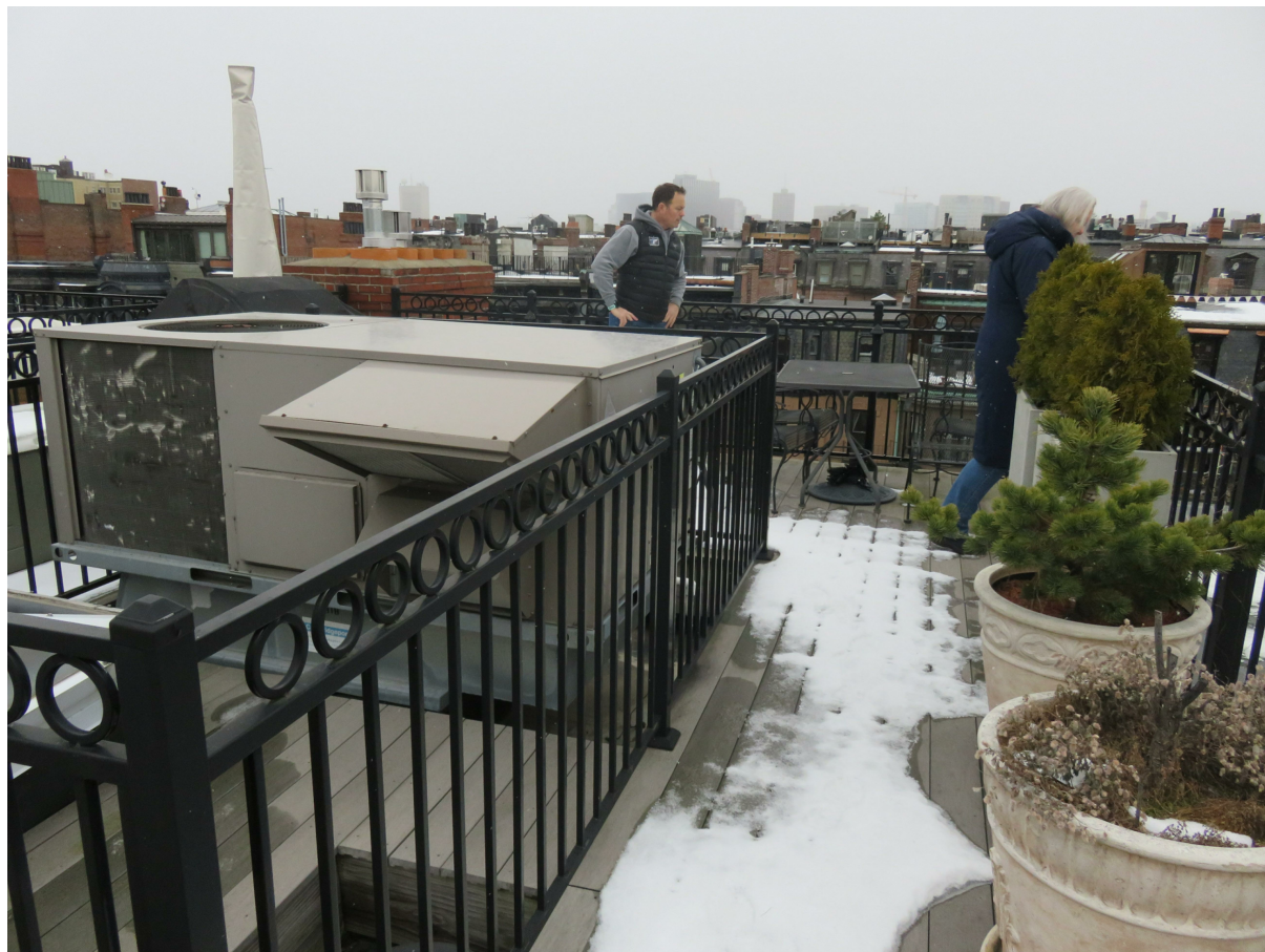
EXISTING ROOF DECK - MECHANICAL
