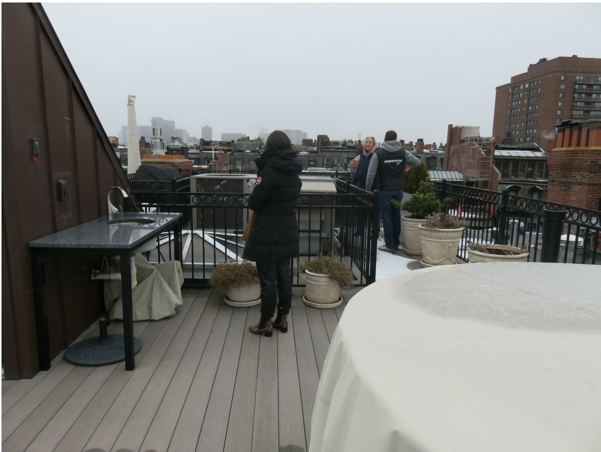
EXISTING ROOF DECK - SKYLIGHT
