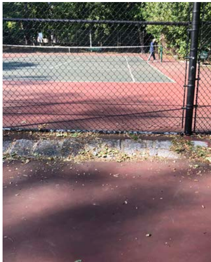
TENNIS COURT FENCE
