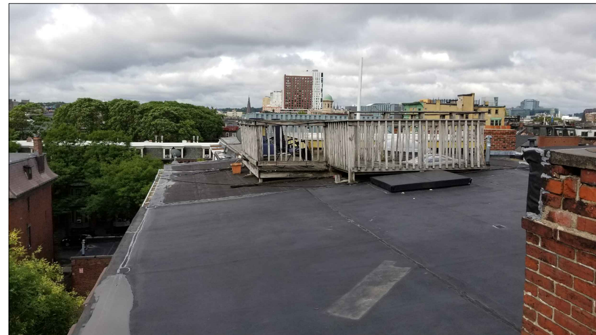
4 ROOF DECK ON ADJACENT BUILDING
