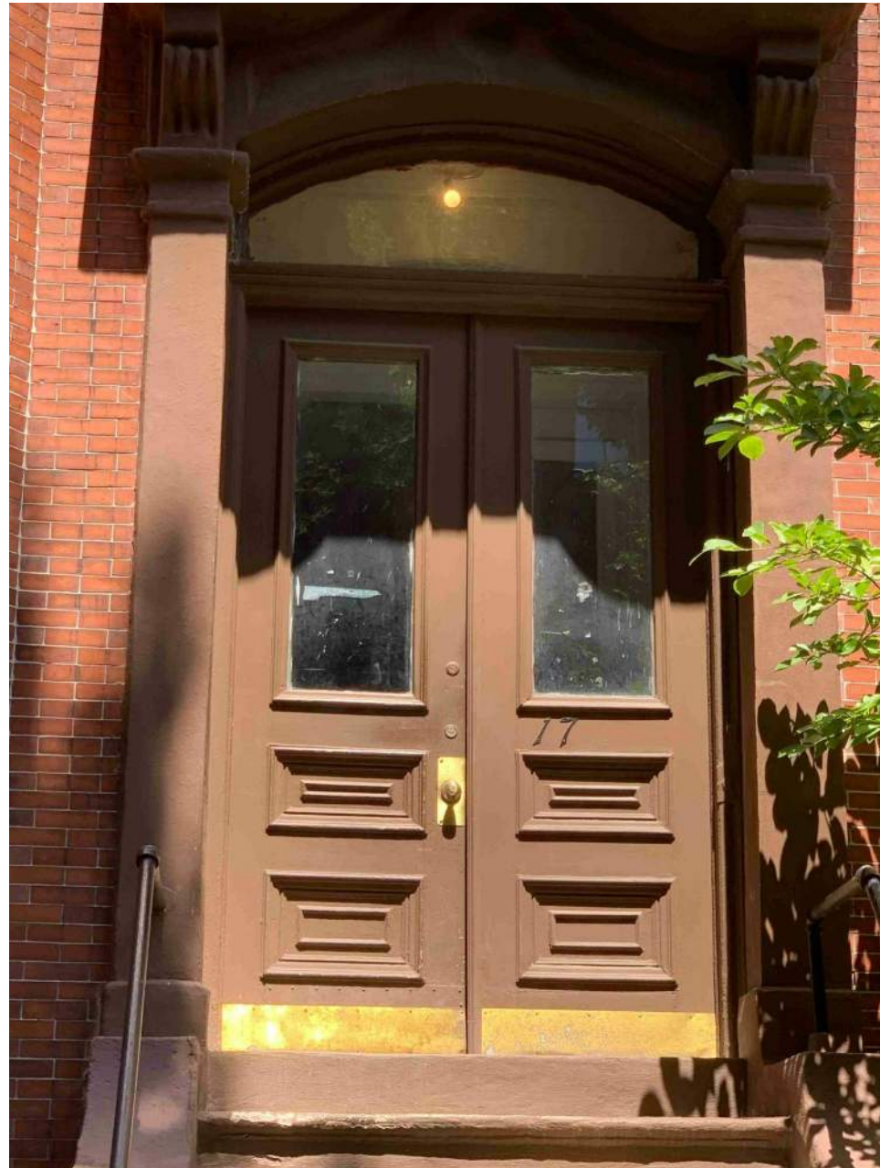
EXISTING DOOR AND HARDWARE
