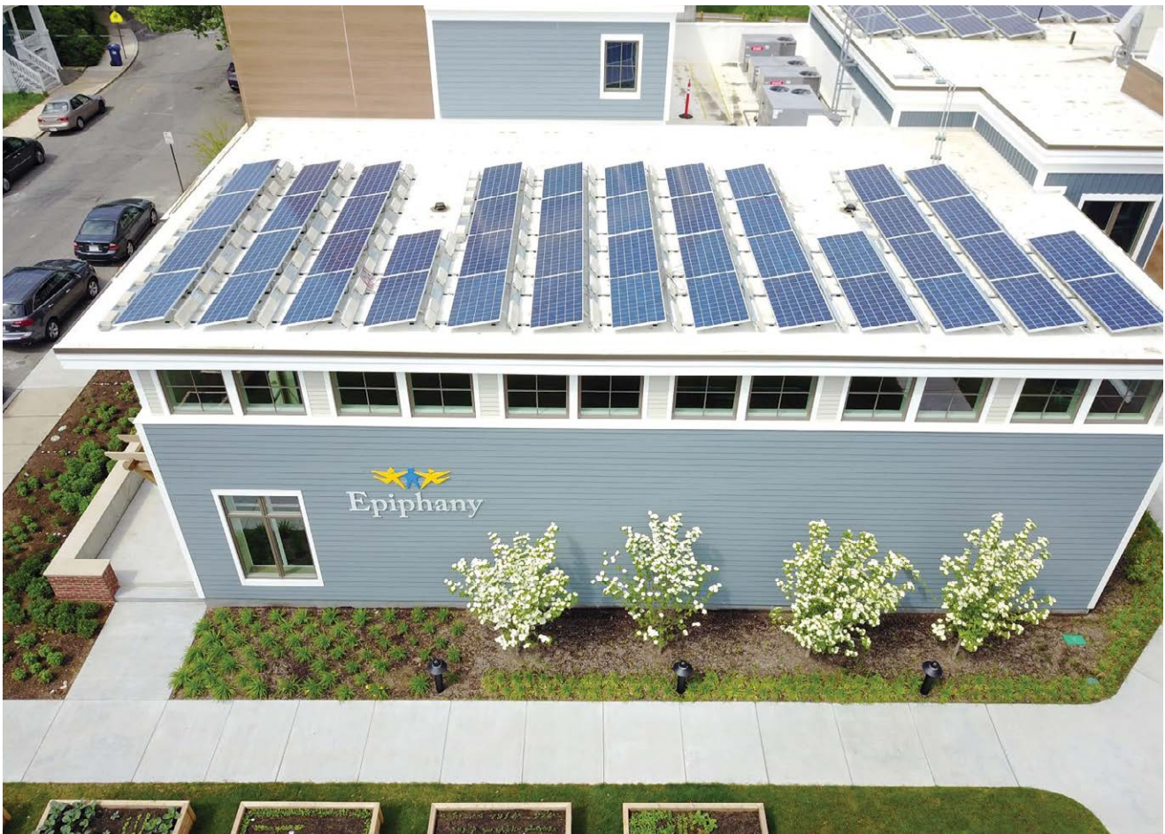
Rooftop solar on the Epiphany School in Dorchester. Photo credit: Resonant Energy
