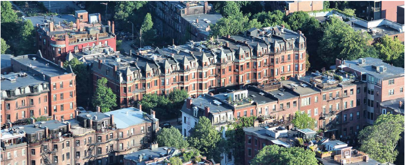
Apartment buildings in Boston's South End neighborhood. Photo credit: Marek Slusarczyk/Alamy Stock Photo
