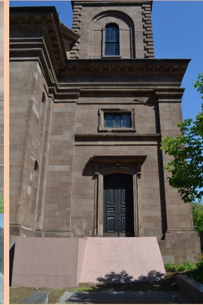
Plywood boxes at south contain the dismantled stairs and stringer
