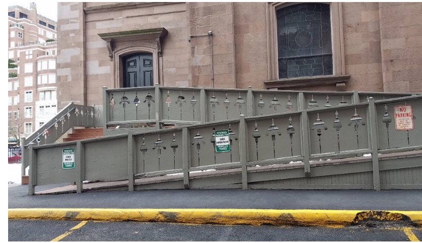
Existing north wood ramp with solid guardrail blocks view of façade.
