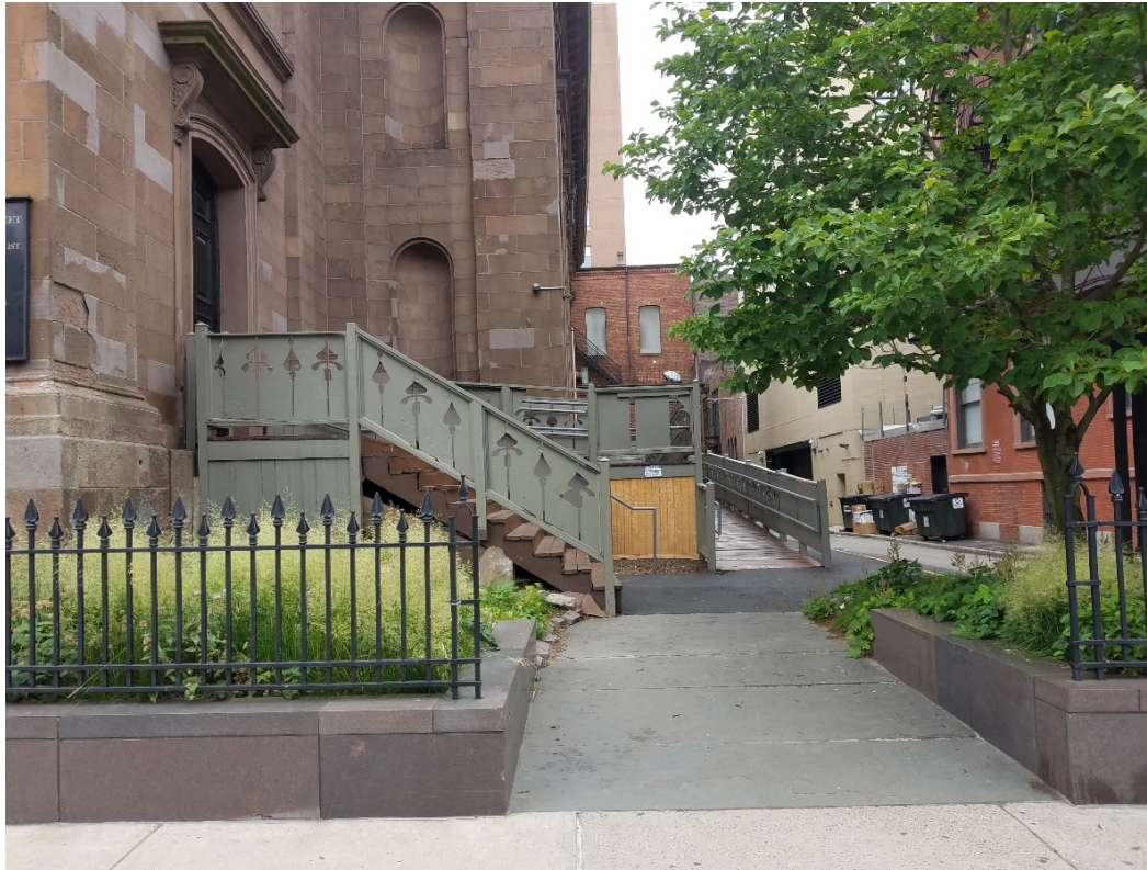
Existing stair and ramp at north
