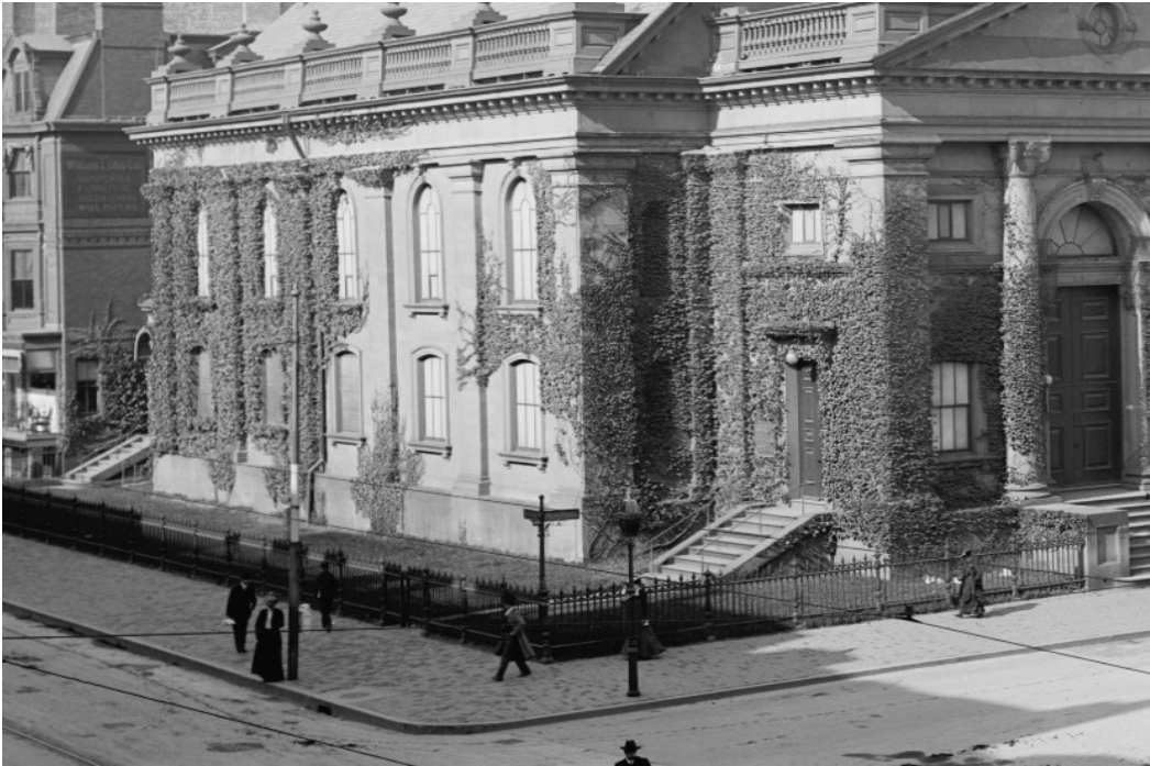
Historic photograph of South elevation
