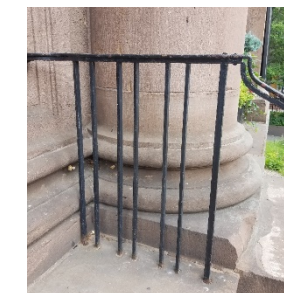
existing paired baluster railing at front entry
