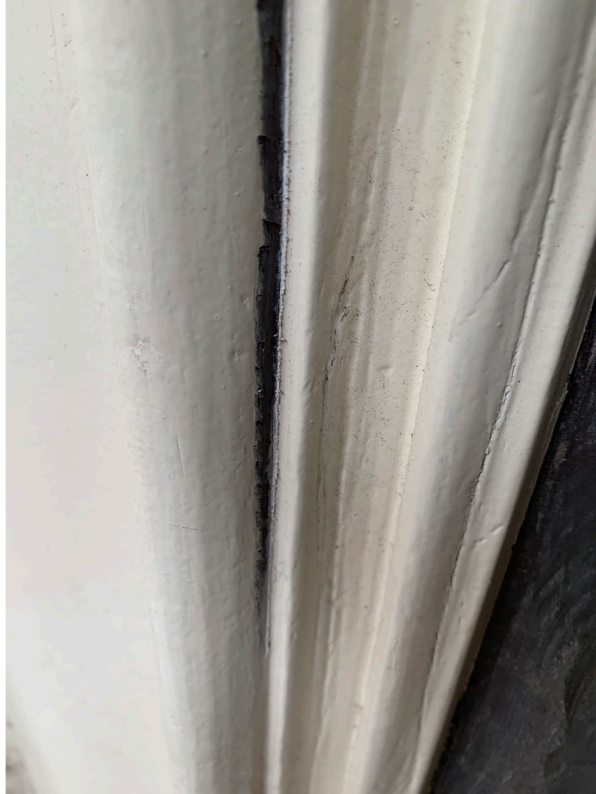
EXPLORATION OF DOOR SURROUND INDICATING BLACK PAINT UNDERNEATH
