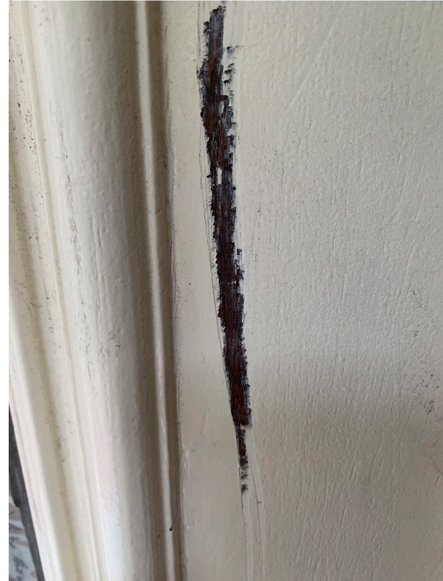
EXPLORATION OF DOOR INDICATING BLACK PAINT UNDERNEATH
