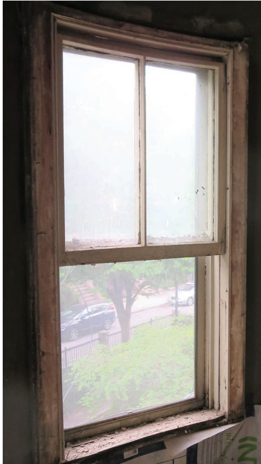
WINDOW 'E' - THIRD FLOOR
