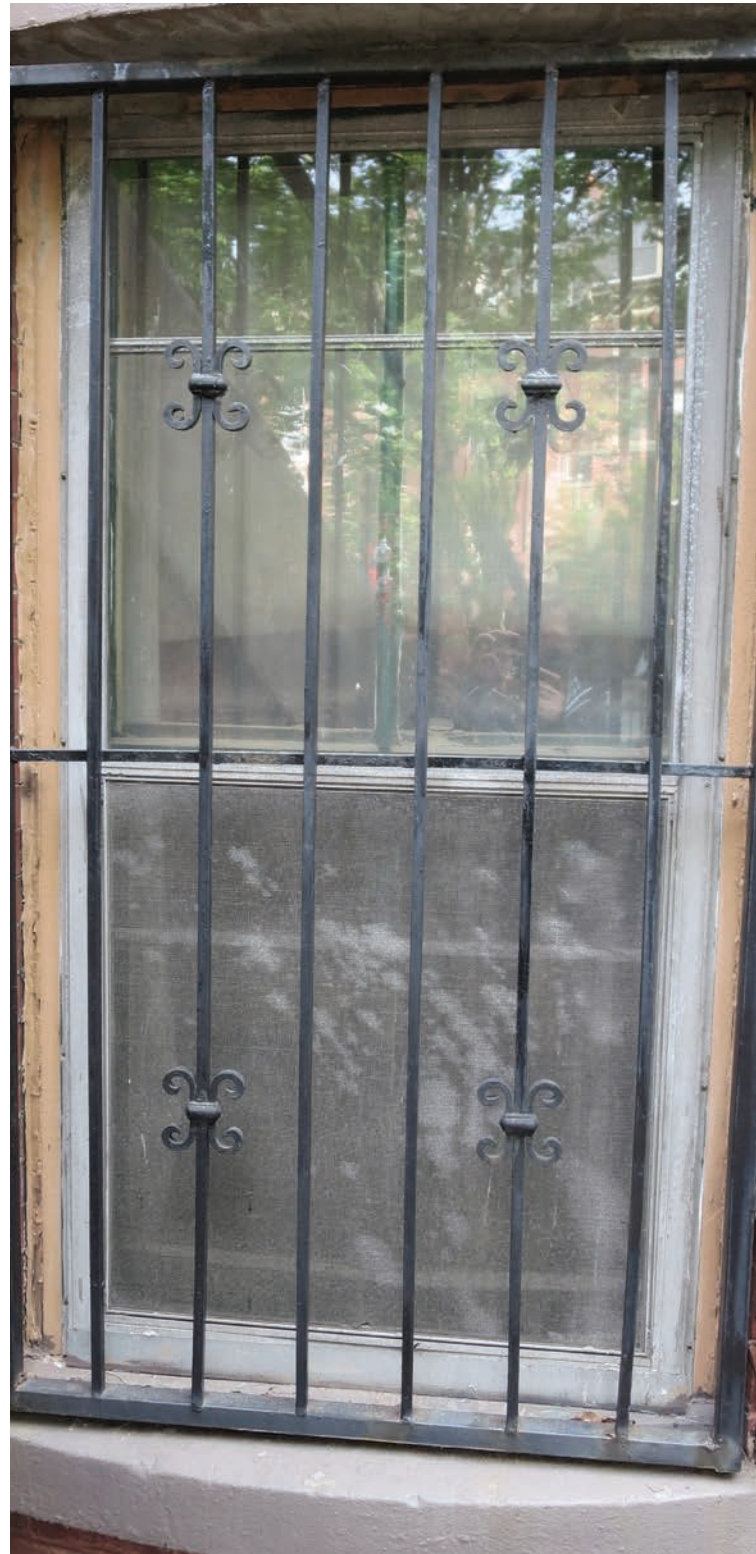
WINDOW 'I' - FIRST FLOOR
