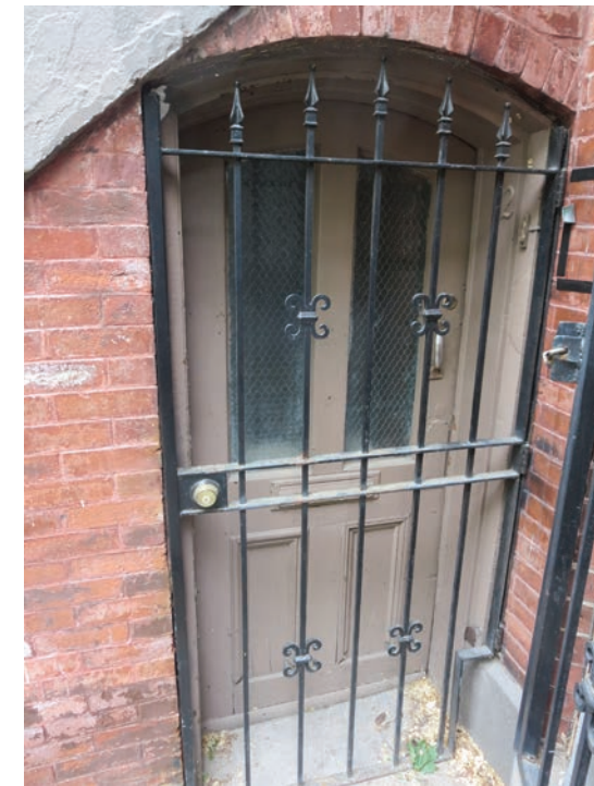
SIDE ENTRY DOOR - FIRST FLOOR
