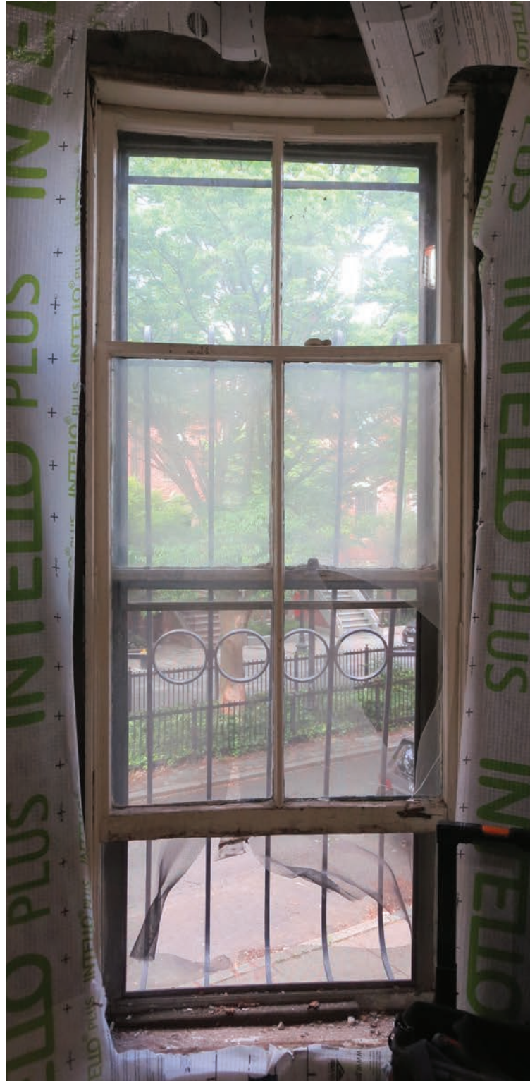
WINDOW 'G' - SECOND FLOOR
