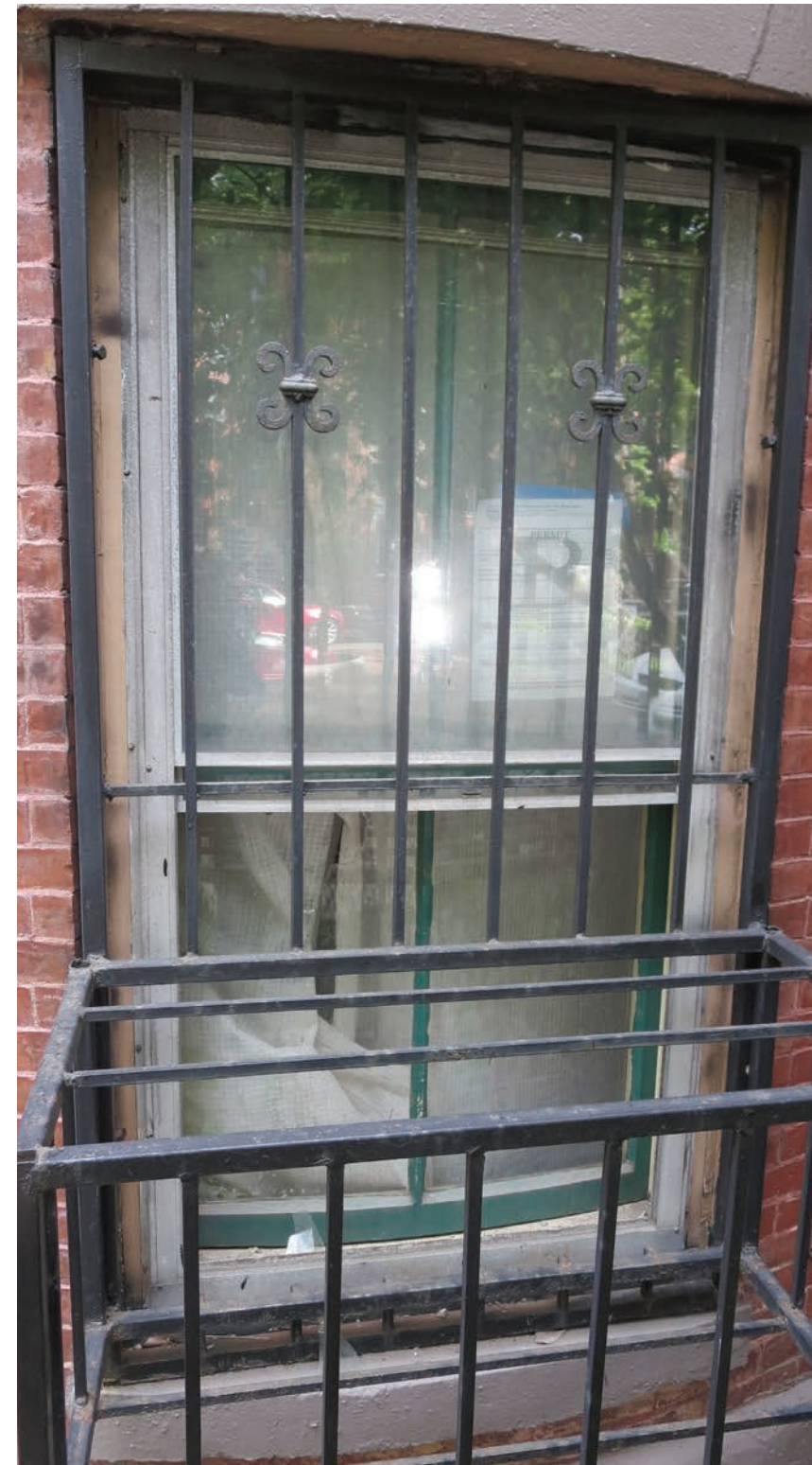
WINDOW 'J' - FIRST FLOOR
