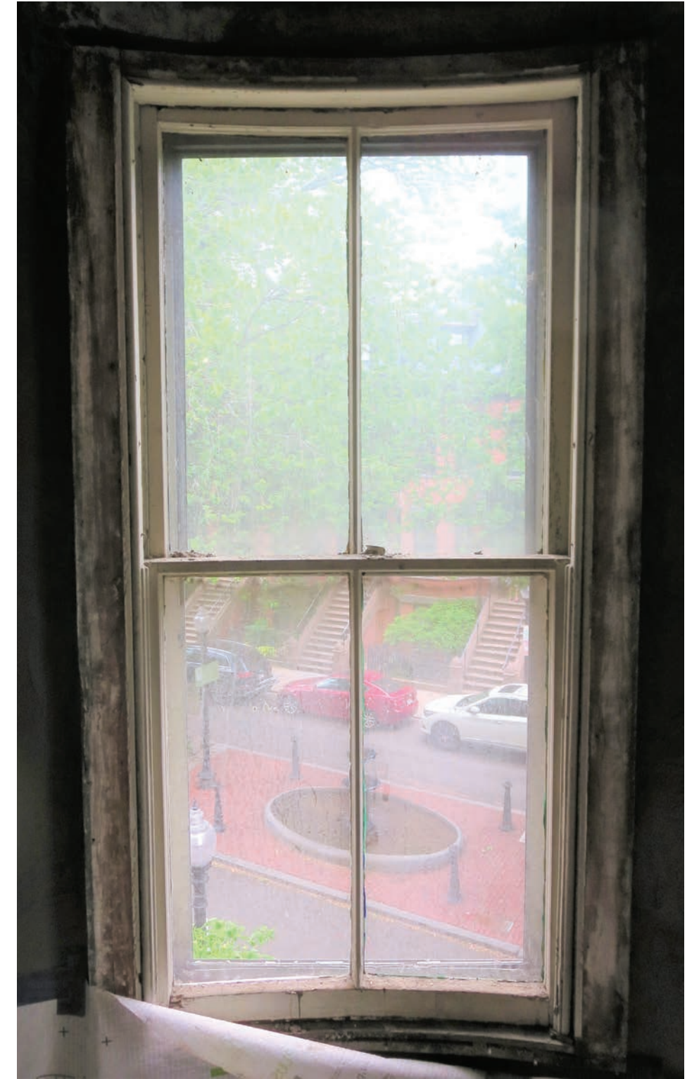
WINDOW 'F' - THIRD FLOOR
