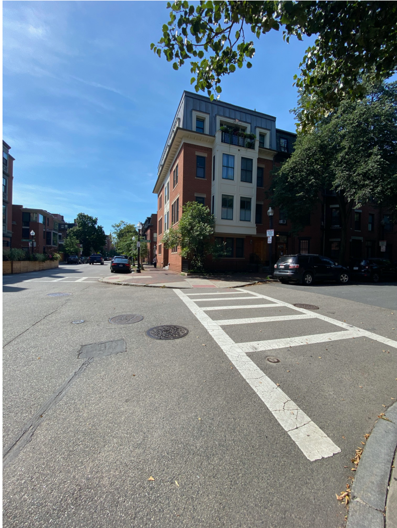
56 Clarendon St – Cross Street Chandler St View
