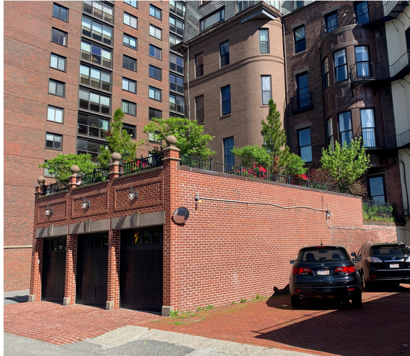
Existing North and West Elevations as seen from Back Street
