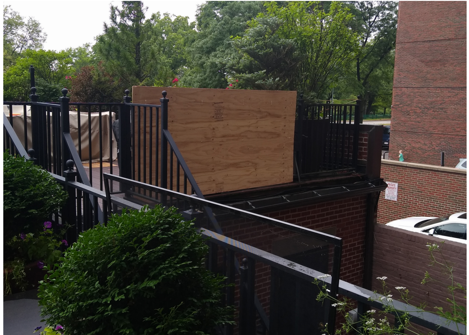
South Elevation from House, with screen wall mock-up located
