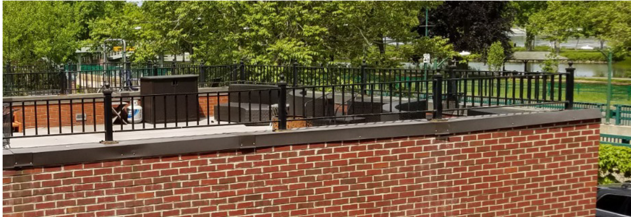
Neighboring deck example of railings installed on parapet wall
