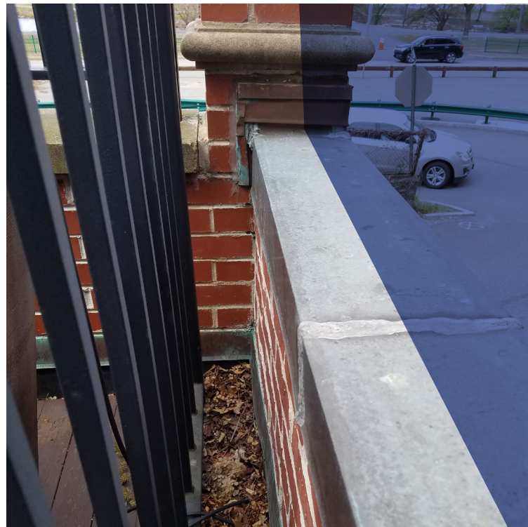
Neighboring deck example of railings installed on parapet wall
