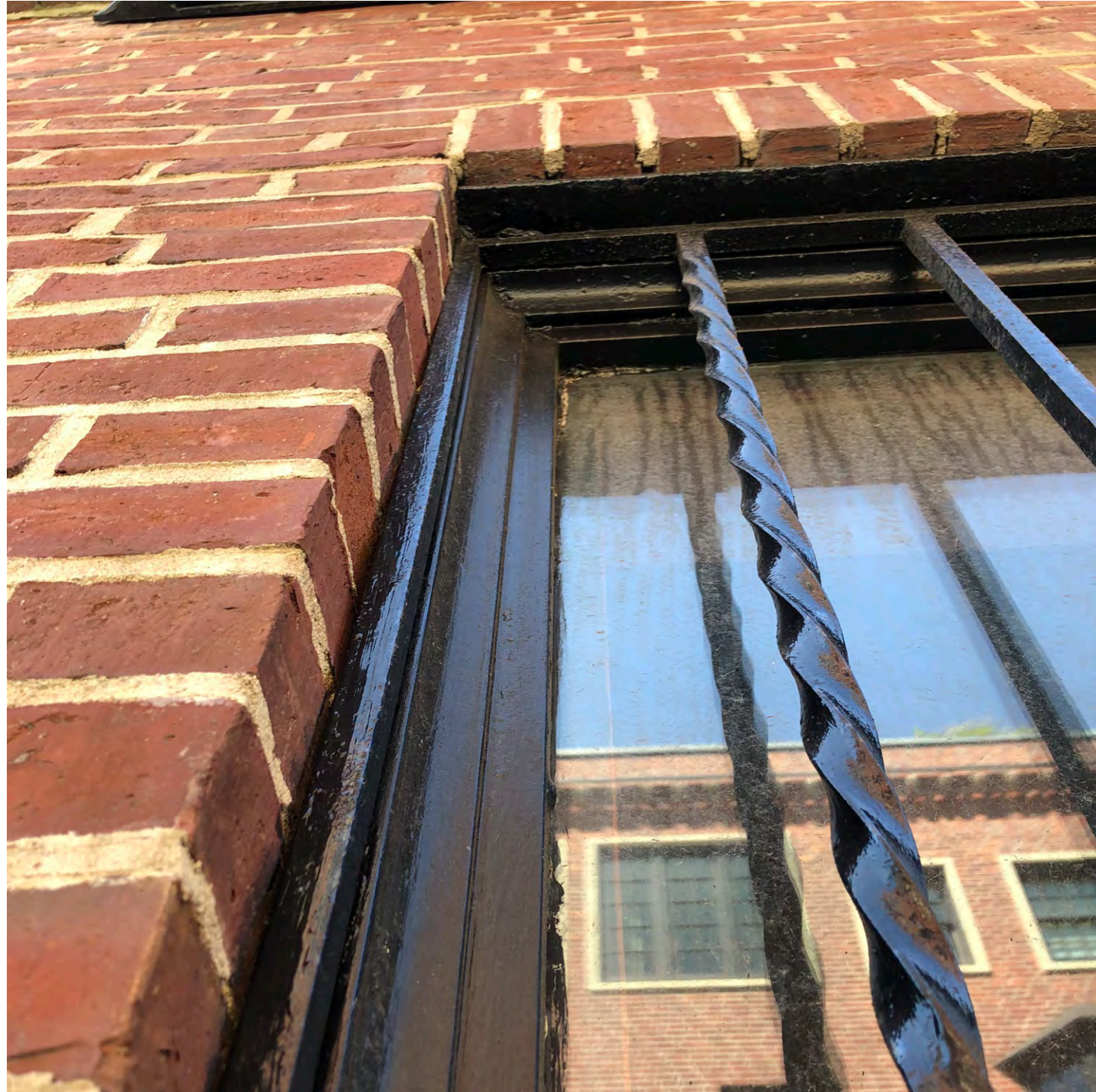
WINDOW C LEFT SIDE HEADER
