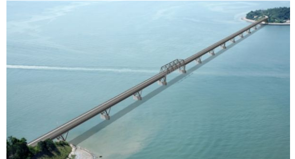
Long Island Bridge
