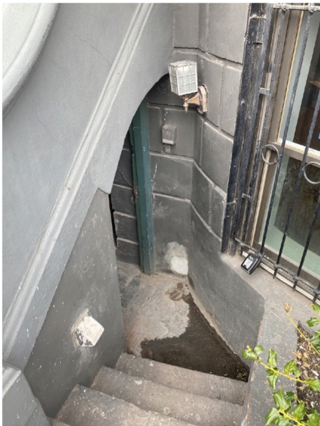
Conditions at 591 Tremont Street
