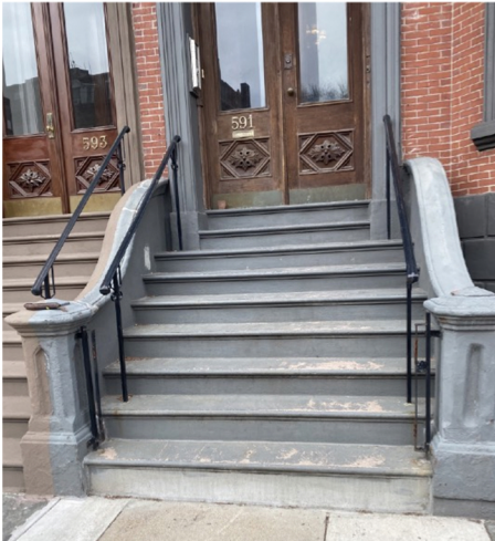
Front steps to be repainted grey
