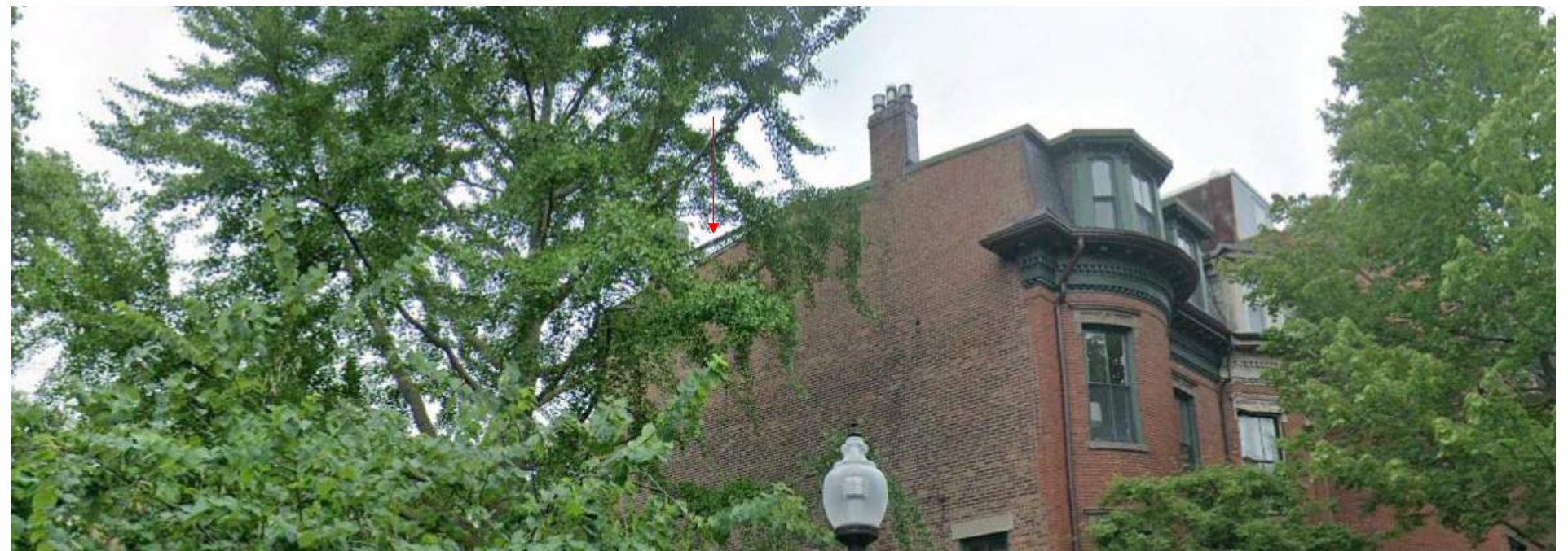
170 West Newton Roof Deck - Viewed from West Newton
