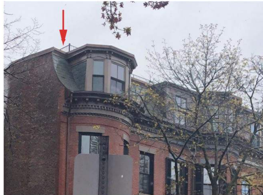
167 West Newton Roof Deck - Viewed from West Newton
