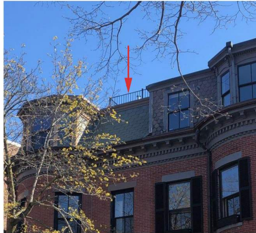
167 West Newton Roof Deck - Viewed from West Newton
