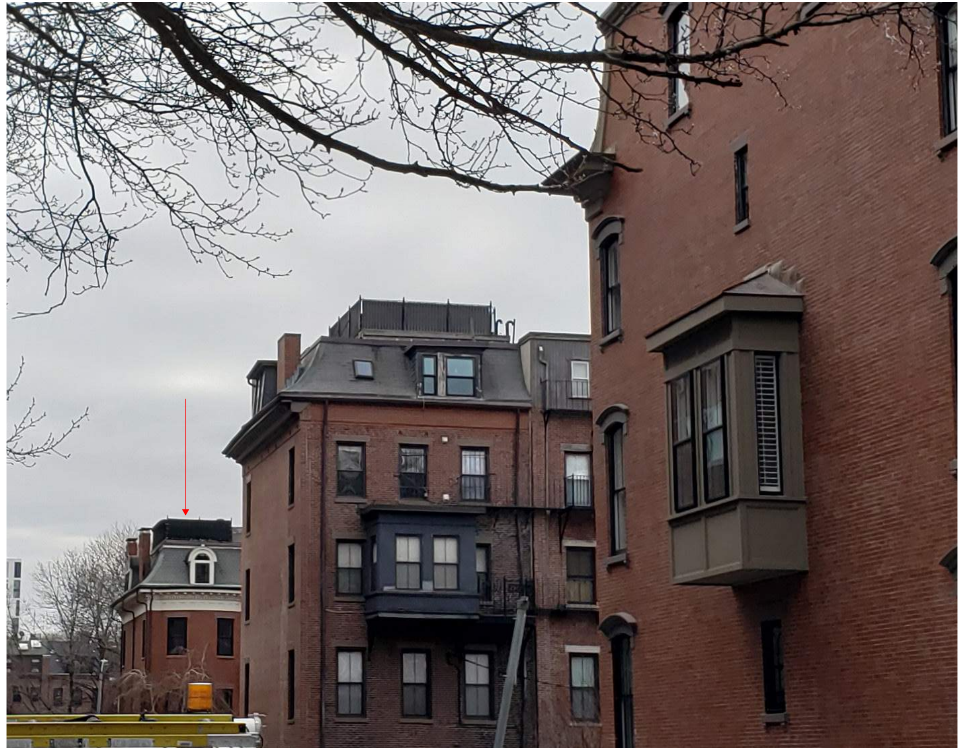
4 Concord Square Roof Deck - Viewed from Rutland Square
