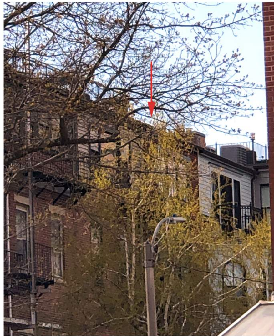
11 Rutland Square Roof Deck Viewed from Tremont St.
