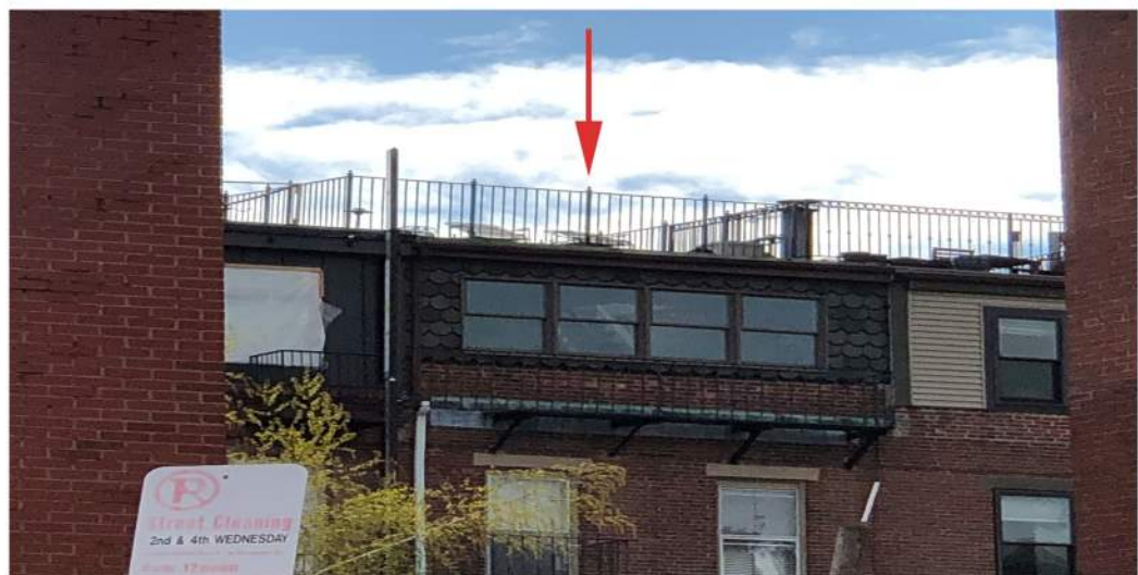
7 Rutland Square Roof Deck - Viewed from West Newton
