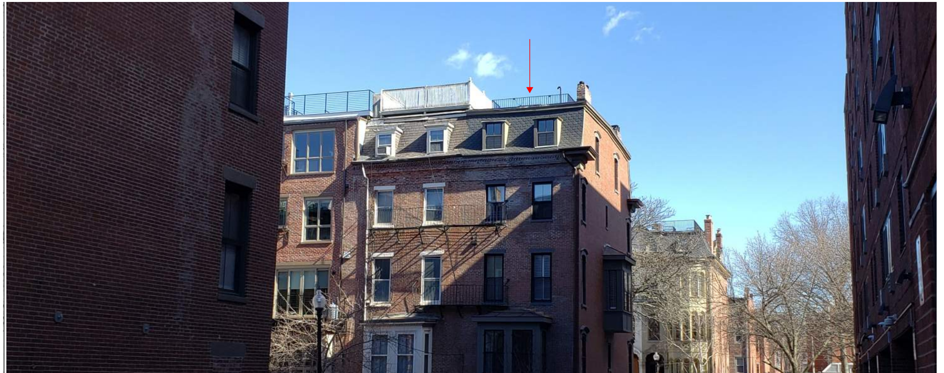
4 Rutland Roofdeck - Viewed from Concord Square
