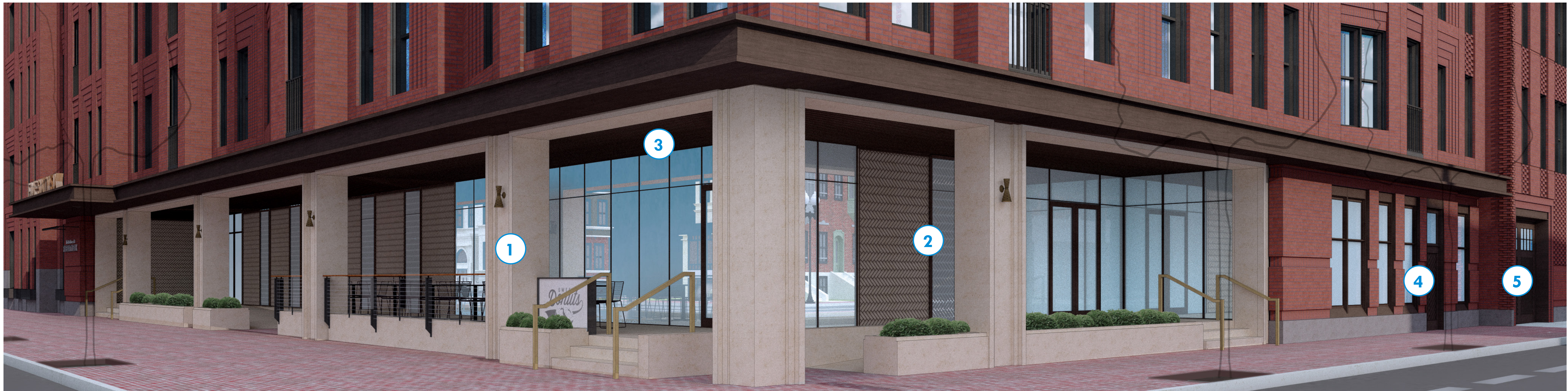
Large format natural stone veneer column enclosures, framed elements and surfaces
