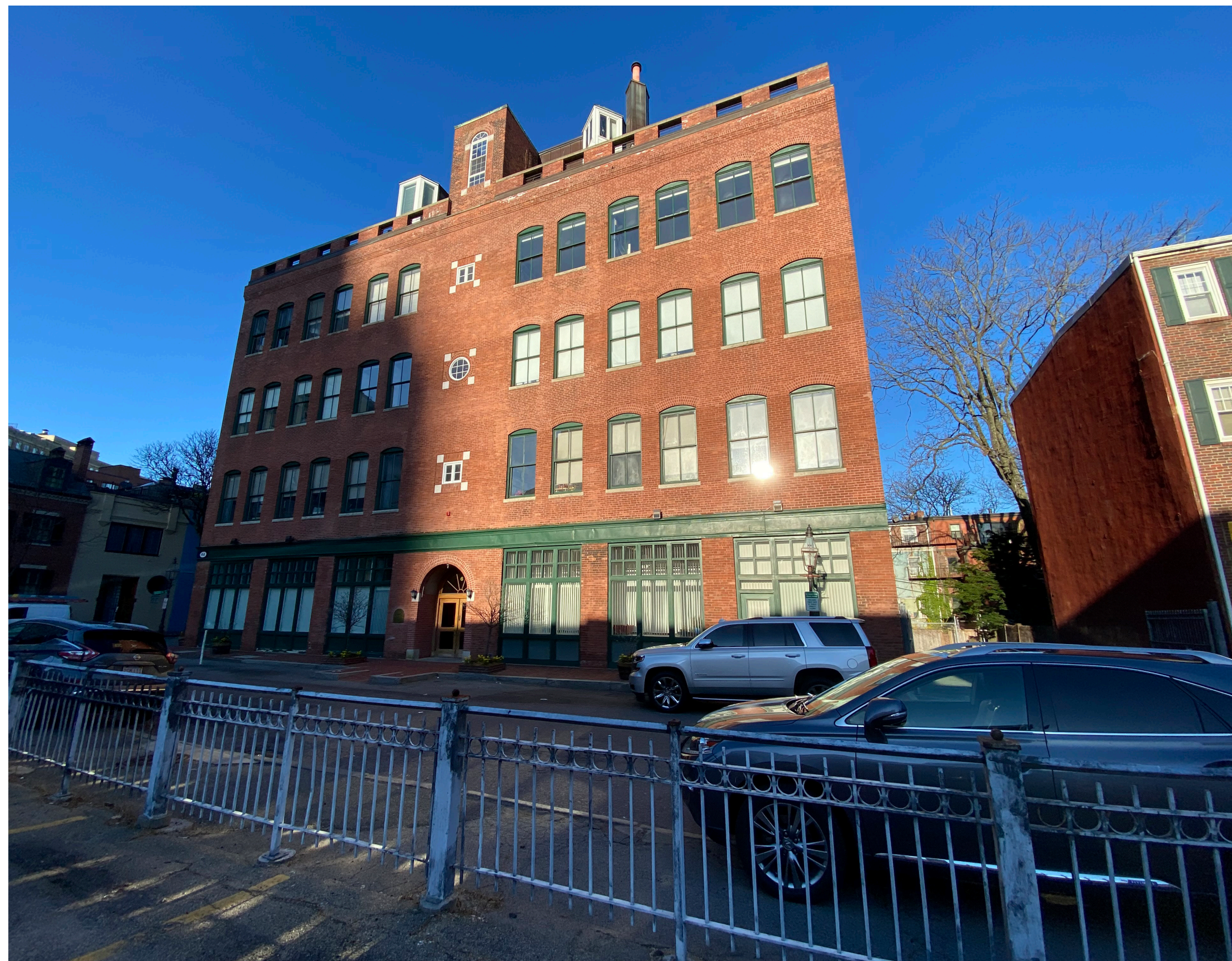
Along Edgerly Place
