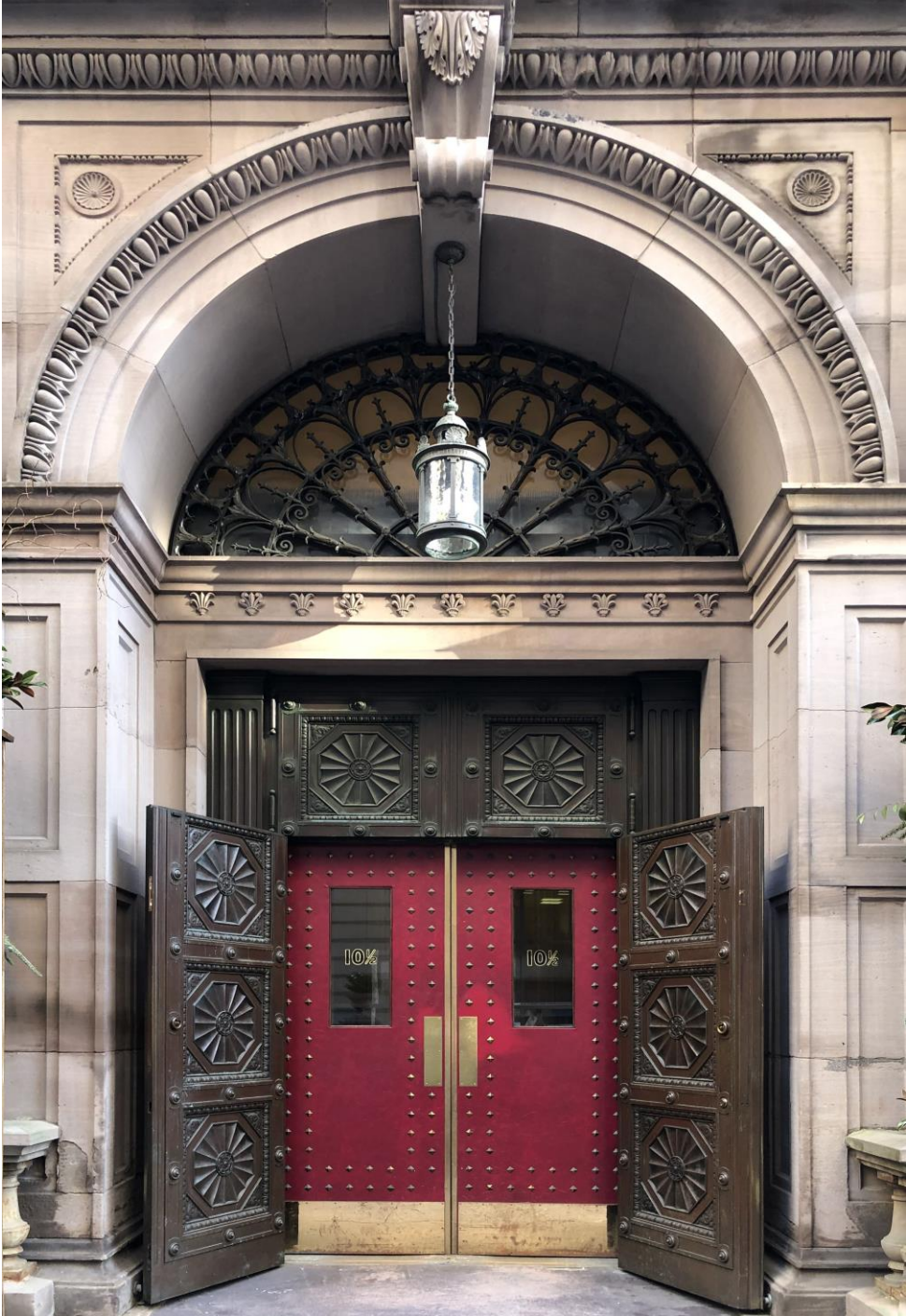
Photo E – Existing Main Entrance Doors
