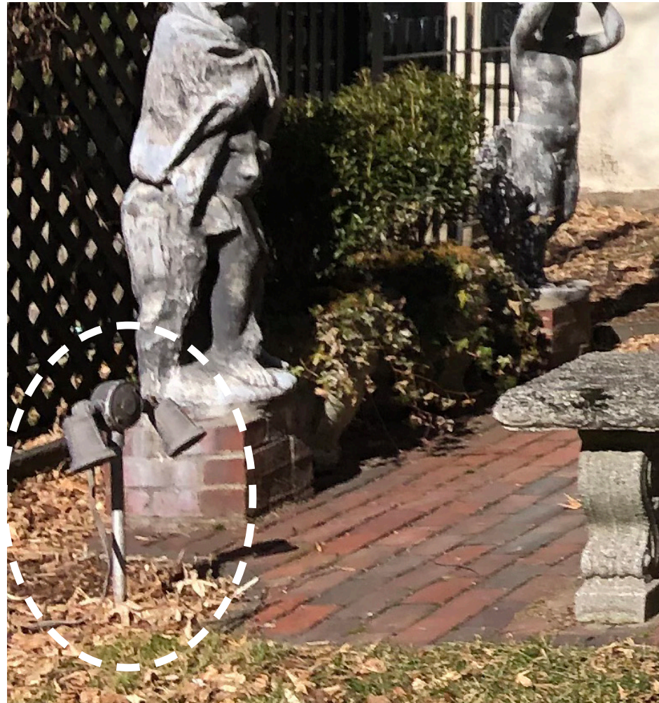
Lighting at the Nichols House Museum, 55 Mount Vernon Street
