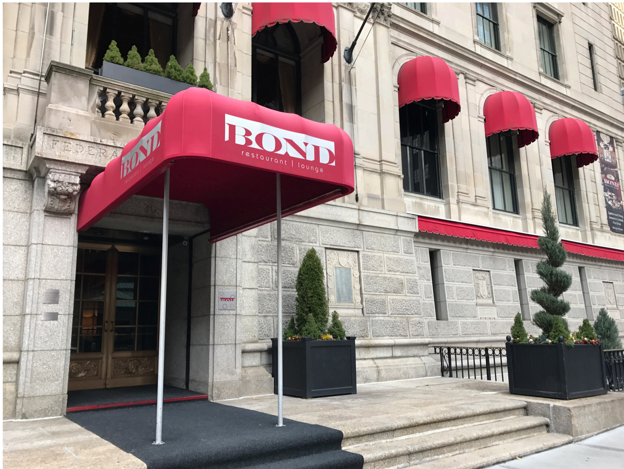
EXISTING PEARL STREET ENTRANCE
