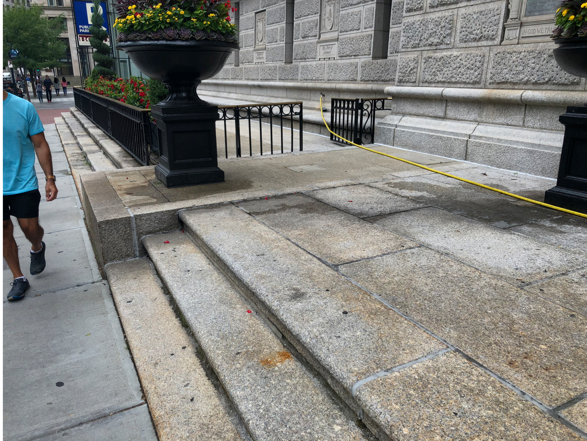
EXISTING PEARL STREET ENTRANCE
