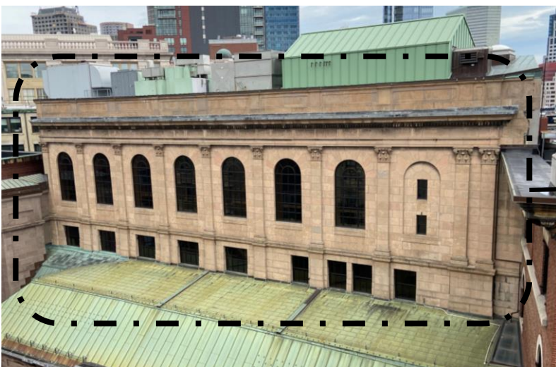
OVERVIEW OF CAST STONE FACADE
