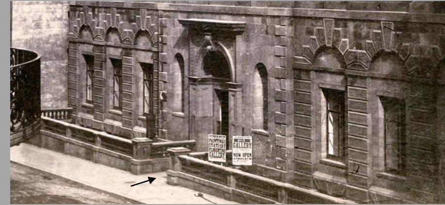
PHOTO 15 – HISTORIC PHOTOGRAPH FROM BOSTON ATHENAEUM WEBSITE INDICATING ORIGINAL LIGHTWELL AND FREE-STANDING PERIMTER WALL. NOTE THAT EXISTING STAIRS (ARROW) NOT PRESENT.
