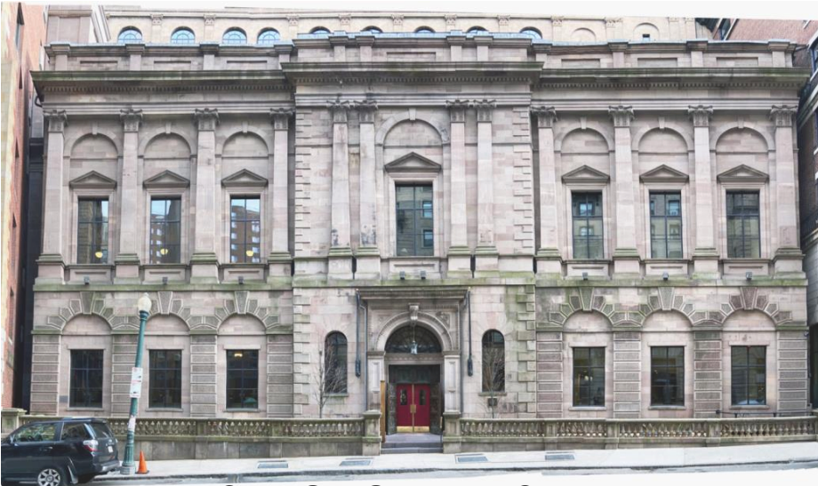
EXISTING NORTH FACADE
