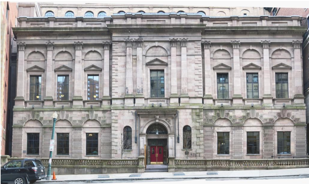
EXISTING CONDITIONS – PHOTOGRAPH OF NORTH ELEVATION
