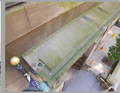
PHOTO 8 – VIEW OF TOPSIDE, UNPROTECTED LEDGE ABOVE MAIN ENTRY.
