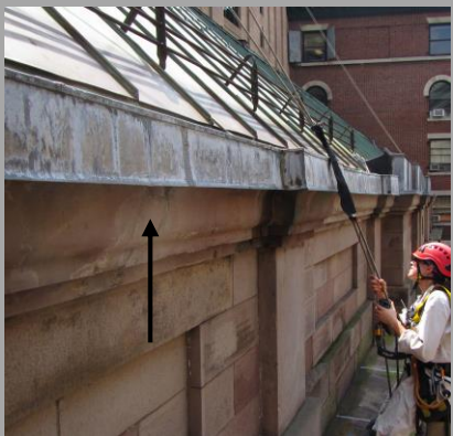
PHOTO 4 – OVERVIEW OF THIRD-FLOOR GUTTER ABOVE MASONRY CORNICE.
