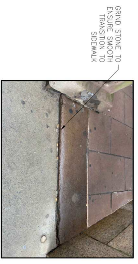
9 STONE GRINDING AT HANDICAP ENTRANCE N.T.S.
