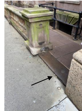
PHOTO 20 – VERTICAL OFFSET BETWEEN SIDEWALK AND STONE TREAD (ARROW).
