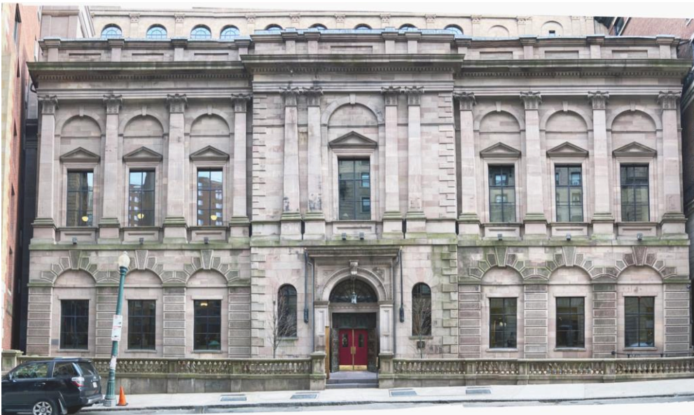
EXISTING CONDITIONS – PHOTOGRAPH OF NORTH ELEVATION
