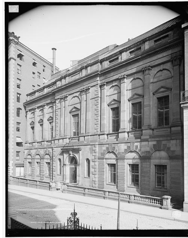
Boston Athenaeum main façade; notable changes that have been made over time include additional two stories, balustrades do not currently wrap towards the door as shown here, addition of basement stair handrail and two flagpoles, currently flank entrance doors in place of this large projecting banner pole; 1906. source: Picryl
