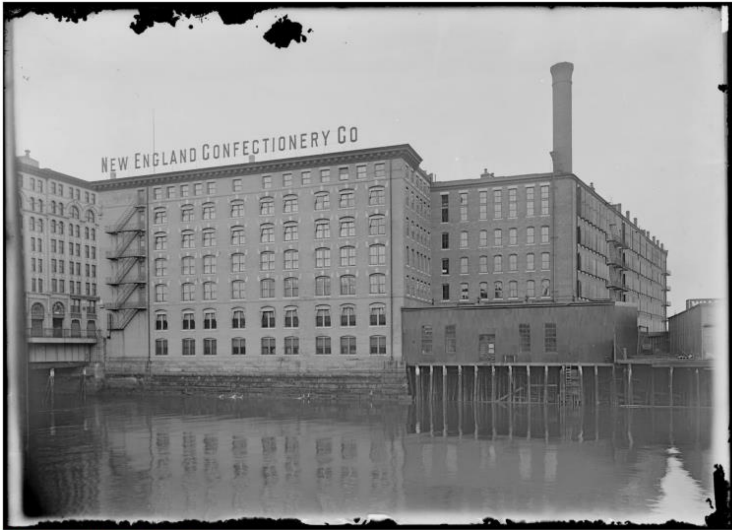
1898-1907 View of 253 Summer Street from Canal
