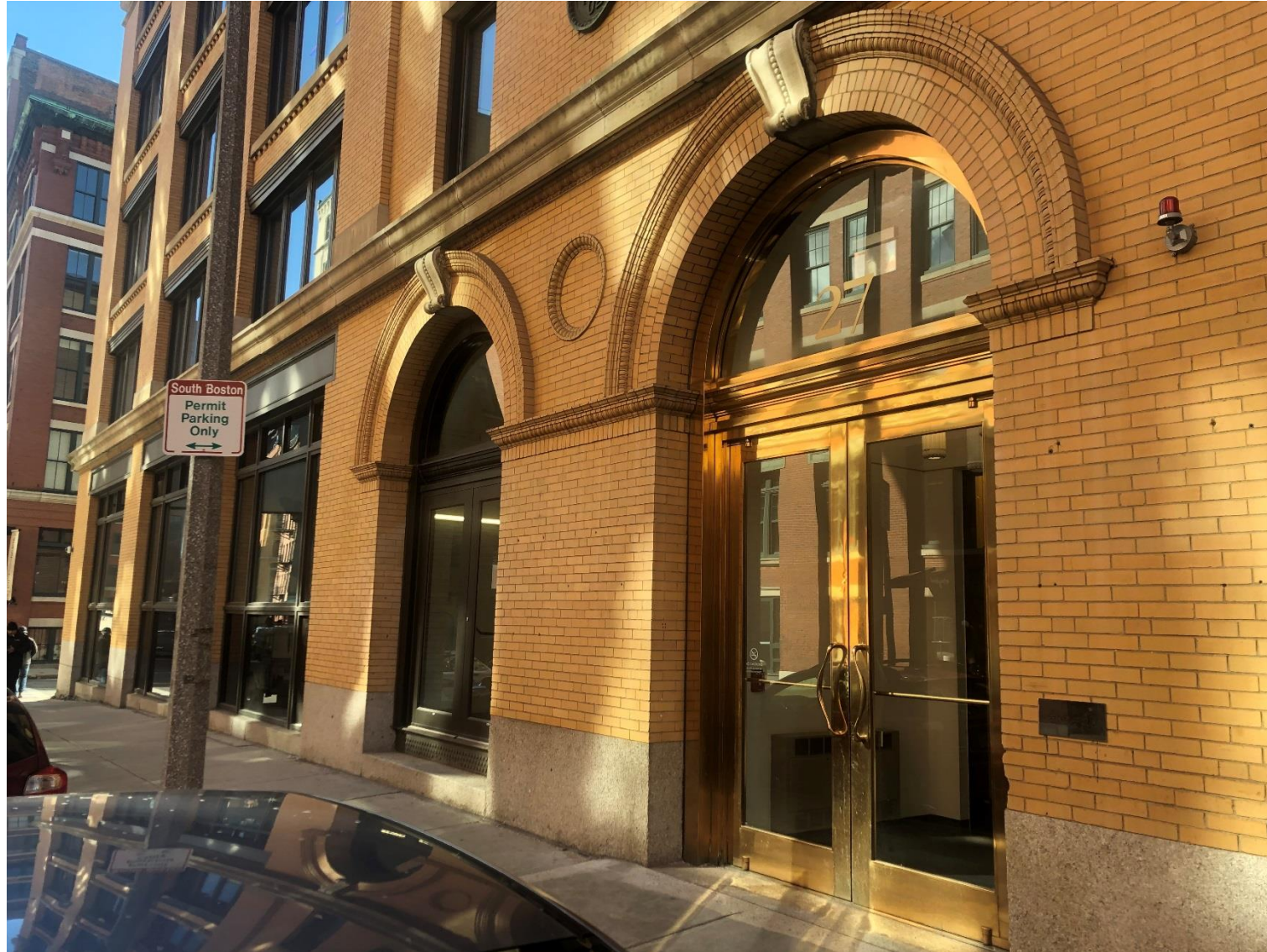
Existing brass clad entry doors shown at right, Feb.,2020
