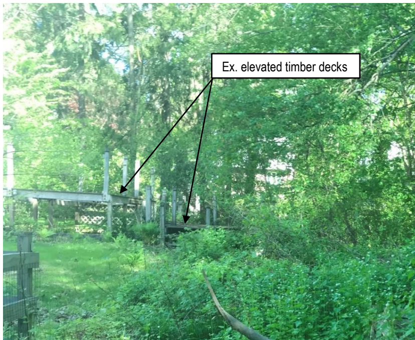
Photograph 3: View (looking east) of the existing elevated timber deck structures located in the backyard. Both structures will be removed as part of the proposed project.
