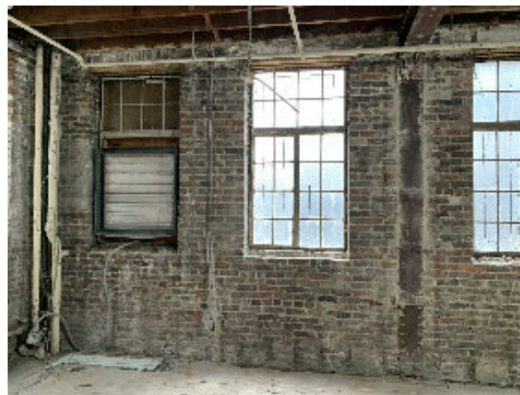
LOT LINE WINDOW VIEW FROM INSIDE
