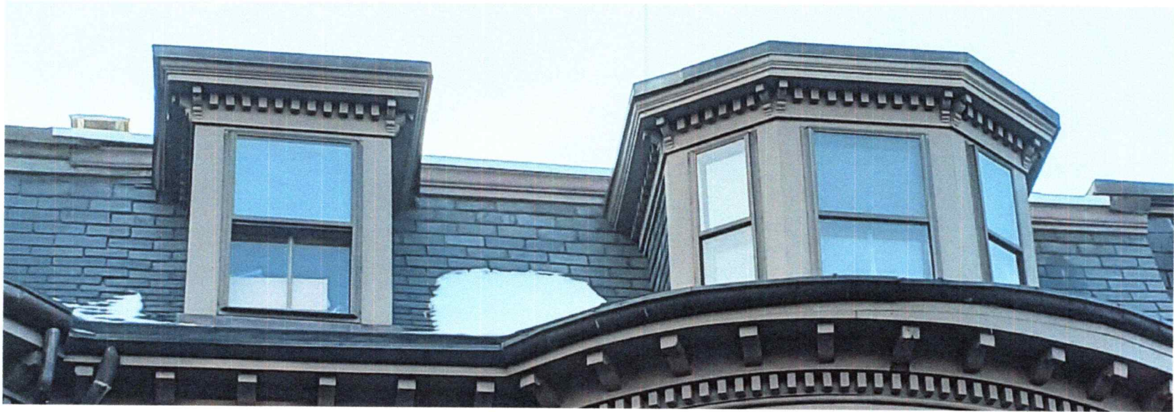
Windows to be replaced, exterior view
