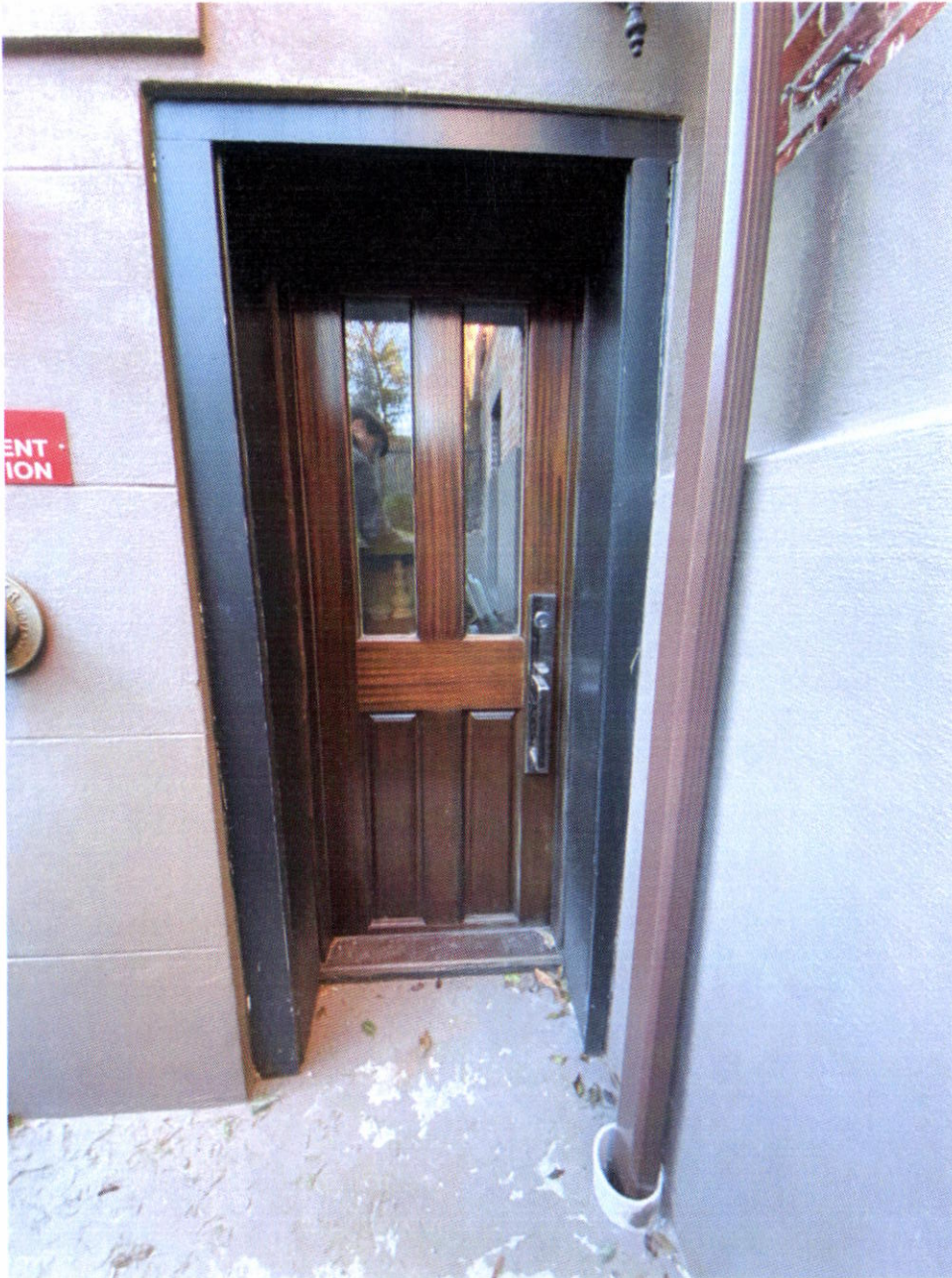
Existing door at 287 Shawmut Ave
