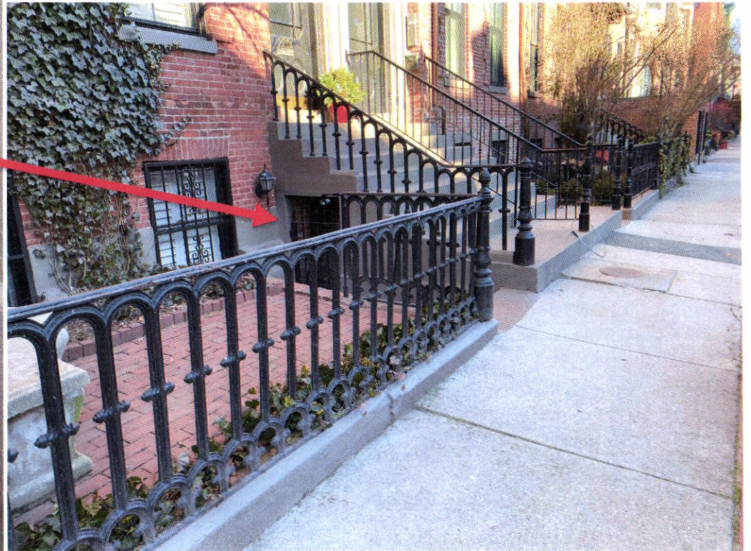
View from sidewalk of current metal security gate
