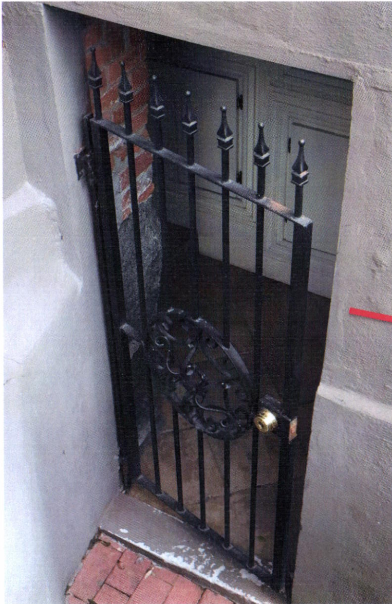
Current installed metal security gate
