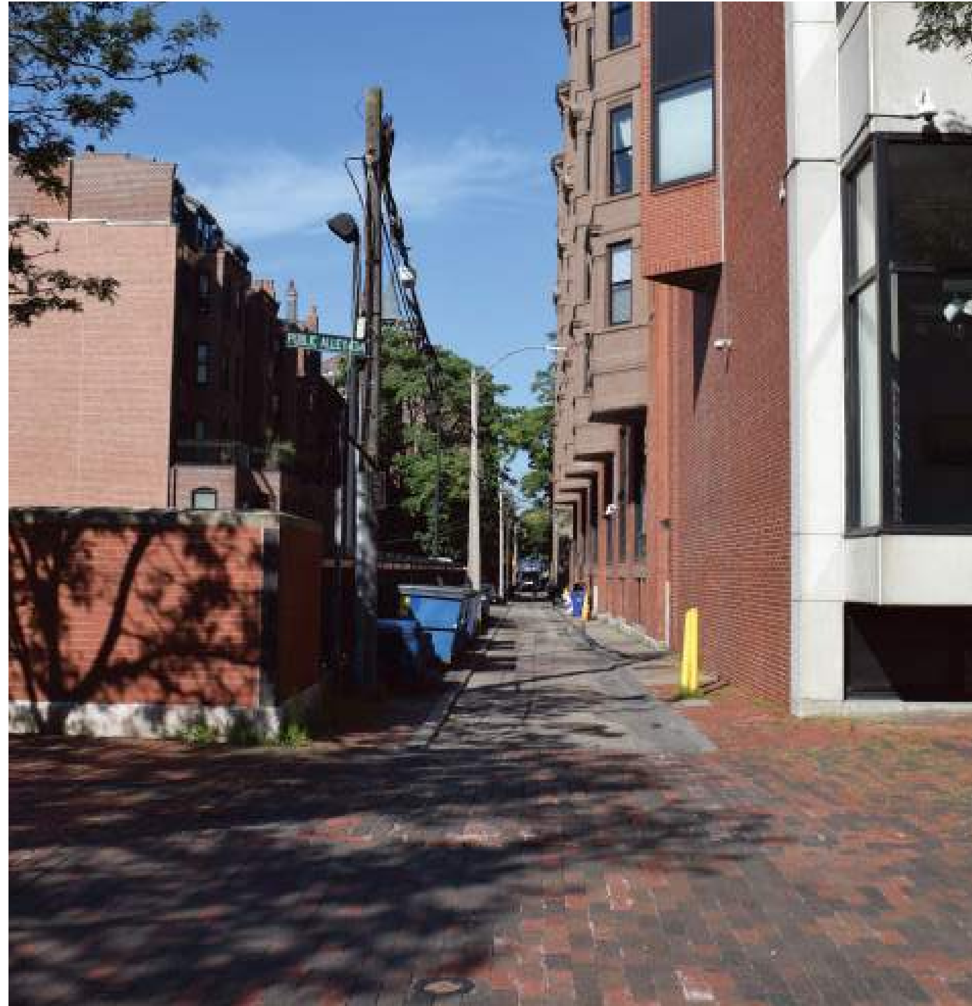
PUBLIC ALLEY 434 FACING WEST
