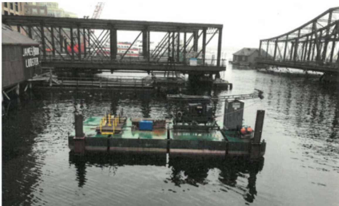
GeoLogic, Inc. Spud-Secured Drilling Barge
