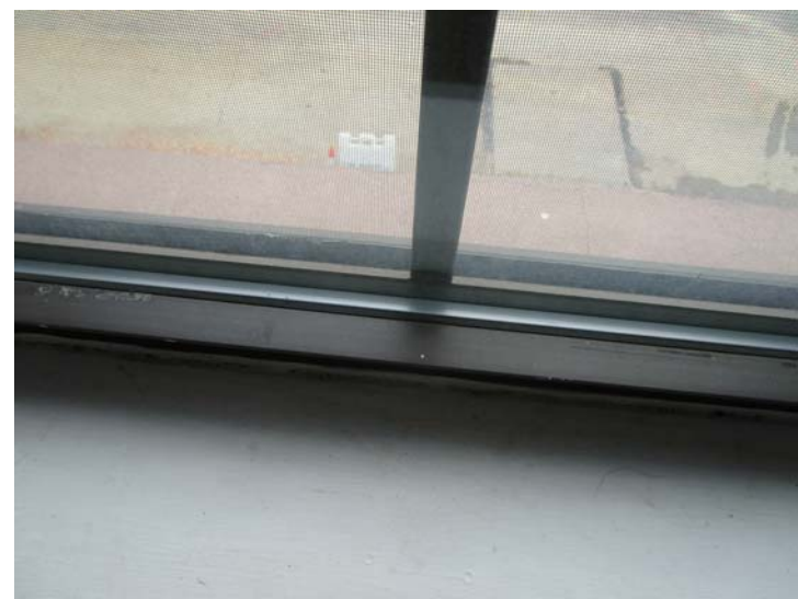
Exterior Muntin from Interior
