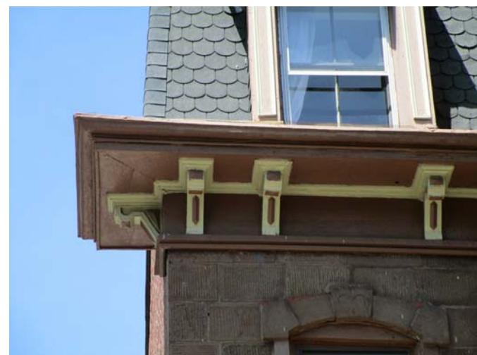
Existing Soffit Details
