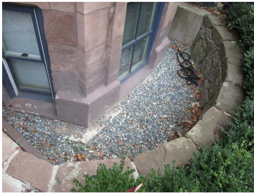
Previously constructed window well 9 Wigglesworth
