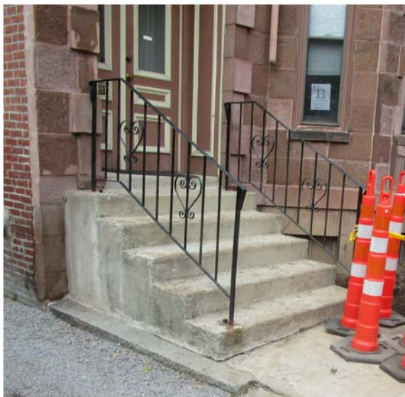
Existing Front Entry Stairs
