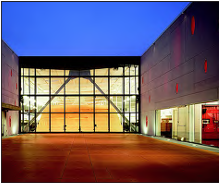
Discreet building mounted floodlighting mounted to upper floors of adjacent buildings
