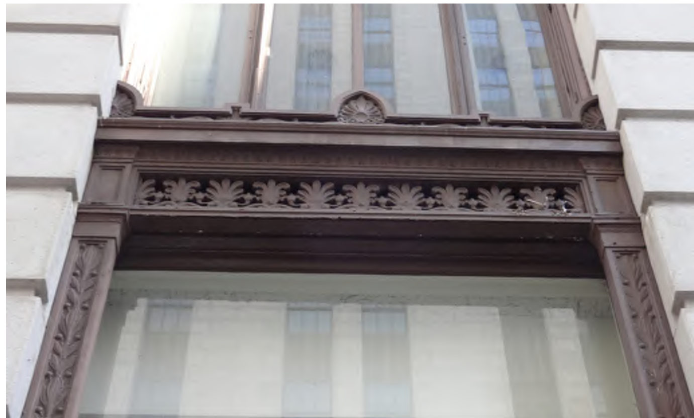
window grillwork detail
