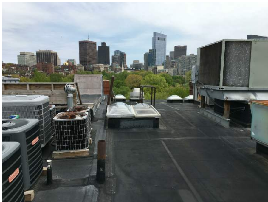
VIEW FROM NW CORNER OF 10-11 ARLINGTON STREET LOOKING EAST
