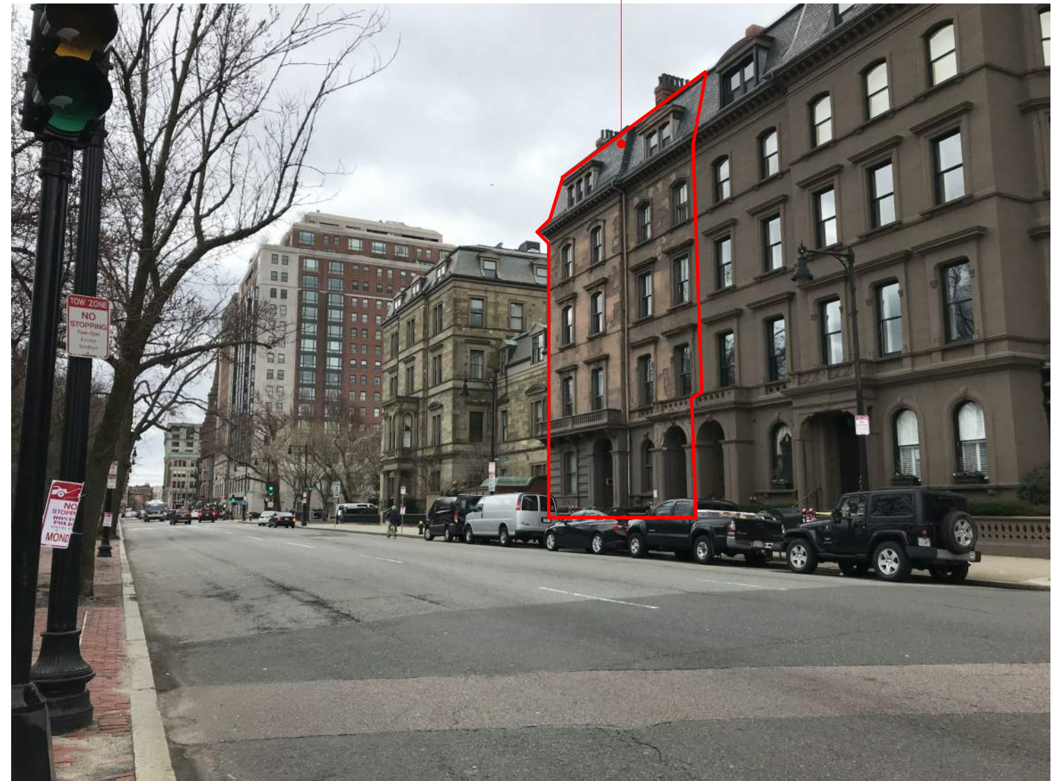
ARLINGTON STREET LOOKING SOUTHEAST
