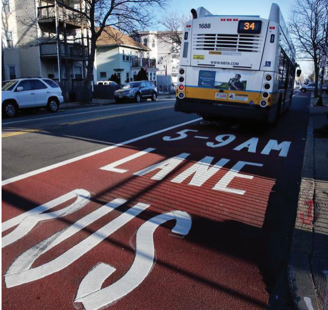
Travel lanes that prioritize buses, like the bus lanes on Washington Street in Roslindale, help ensure faster and more reliable service for riders.
