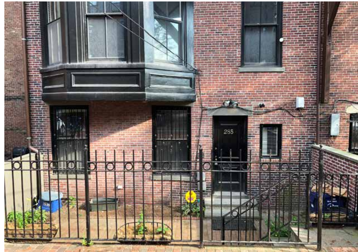
View of Back Patio
