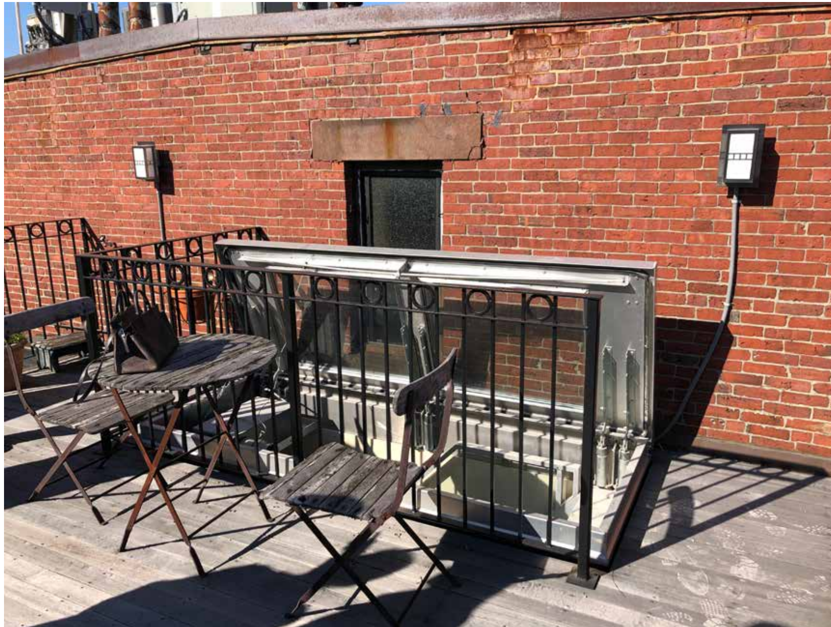
Roof Deck Hatch - Existing Conditions
