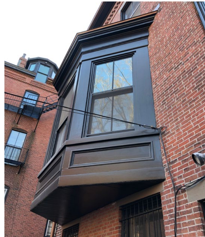
View of Bay Window
