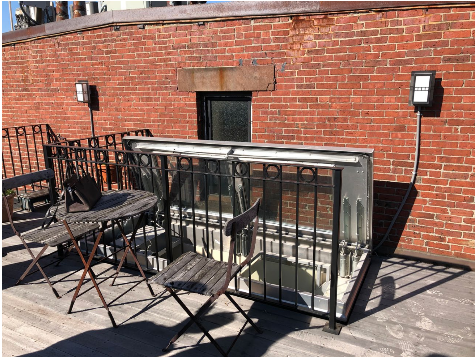
Roof Deck Hatch - Existing Conditions
