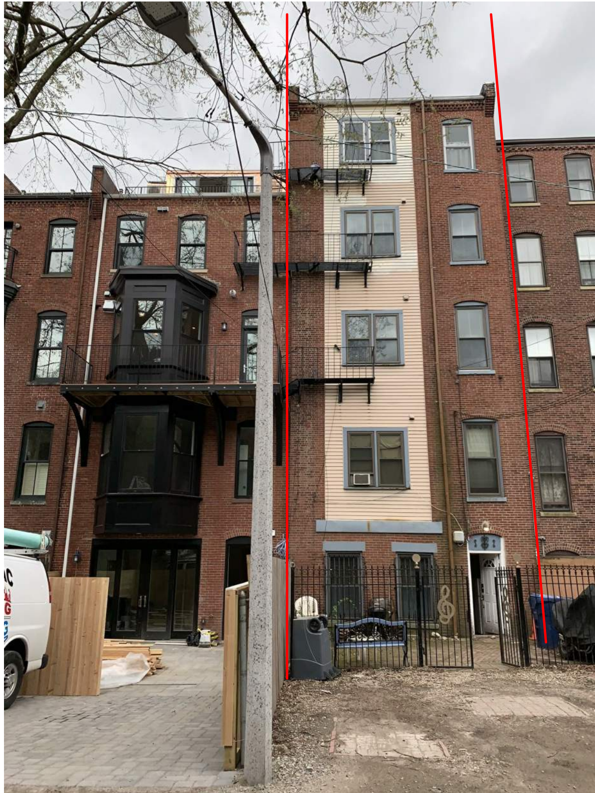
11HF CLAREMONT PARK WITH REAR CHIMNEY VIEW
