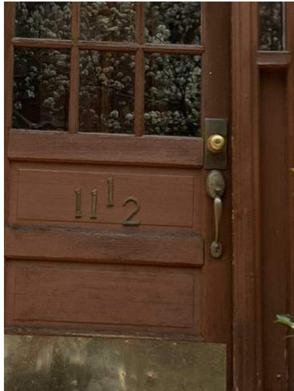
EXISTING DOOR HARDWARE
