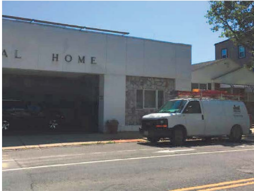
Photo Three Caption NORTH SIDE - CHELSEA STREET 08-26-2019 Clear Photo Three
