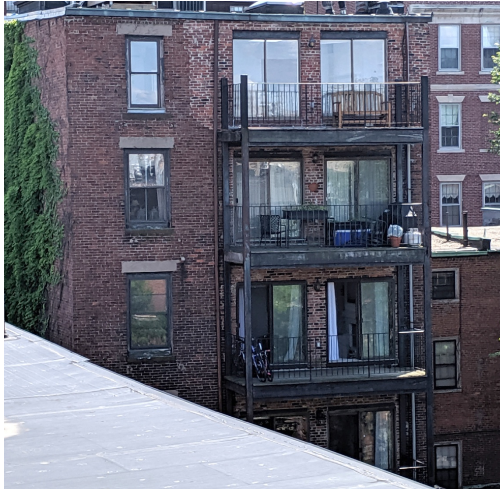
View of 23 Pinckney Street, from another rooftop across Myrtle street.
