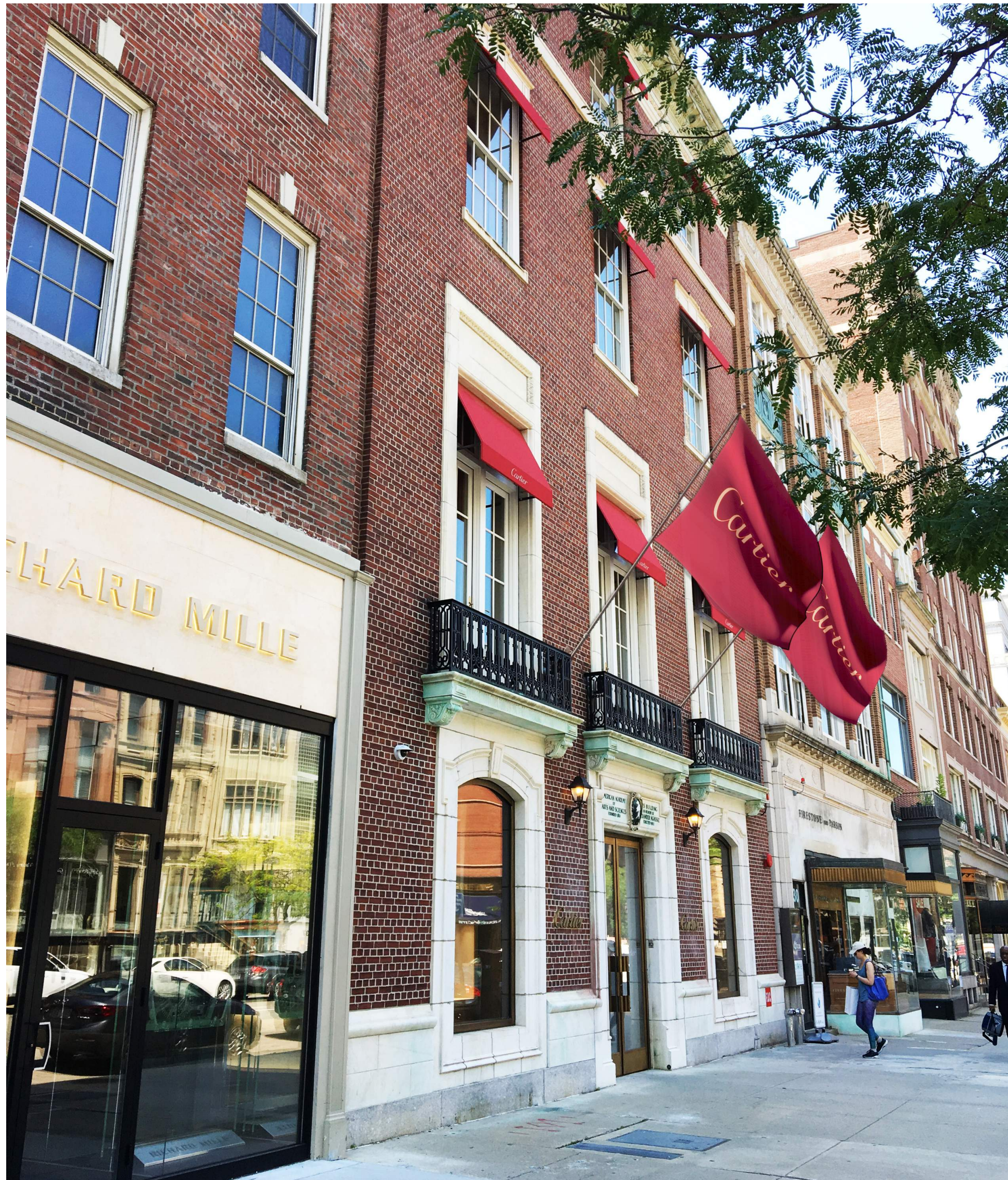
1: VIEW APPROACHING FROM ARLINGTON ST.
