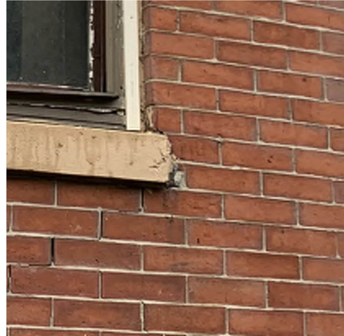
EXISTING SHUTTER DOG HOLES AT 24 UNION PARK
