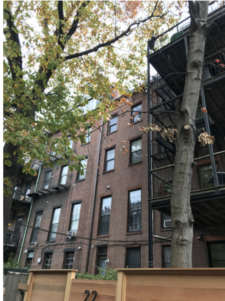
EXISTING REAR VIEW OF CHIMNEY
