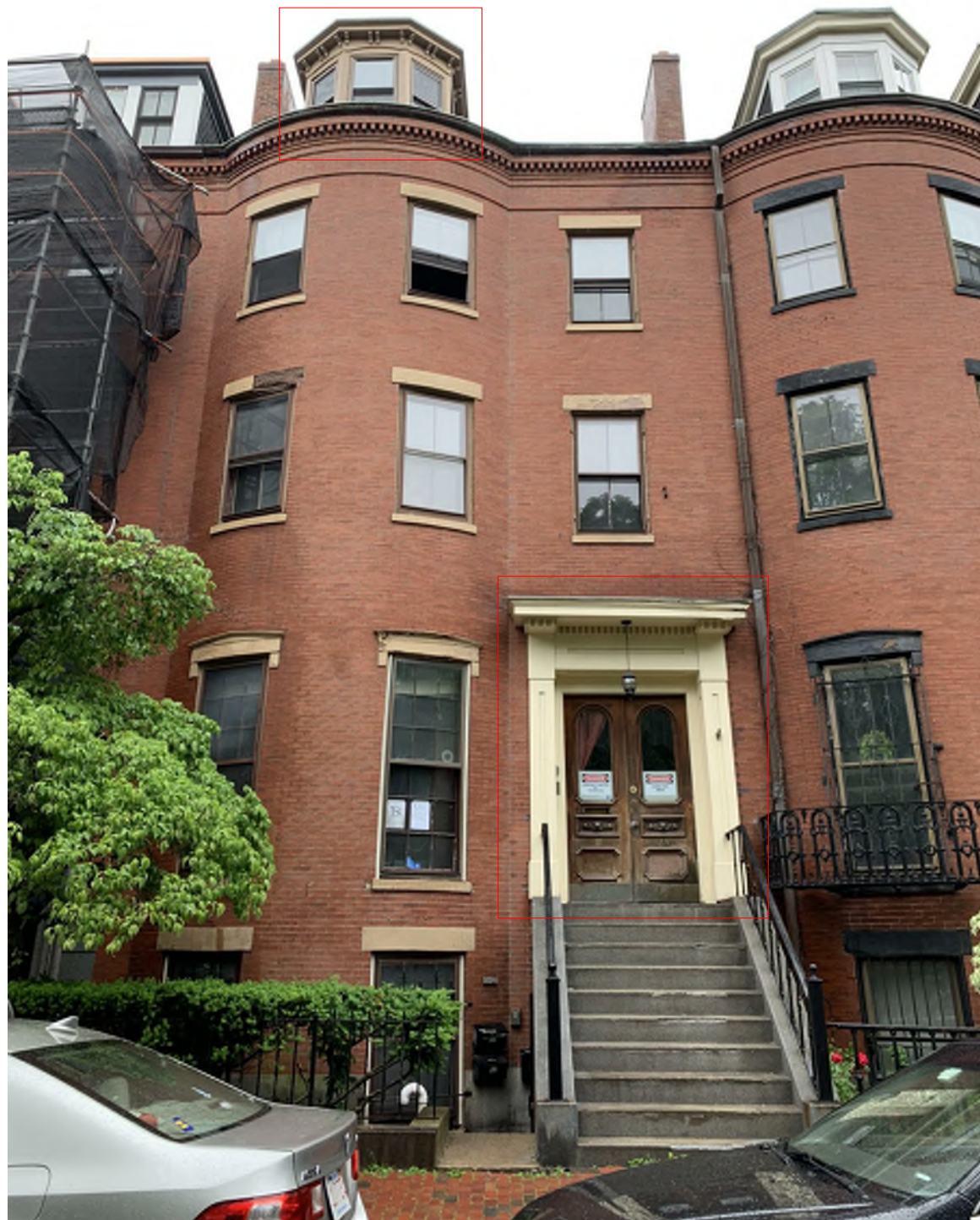
EXISTING FRONT DOOR SURROUND & DORMER
