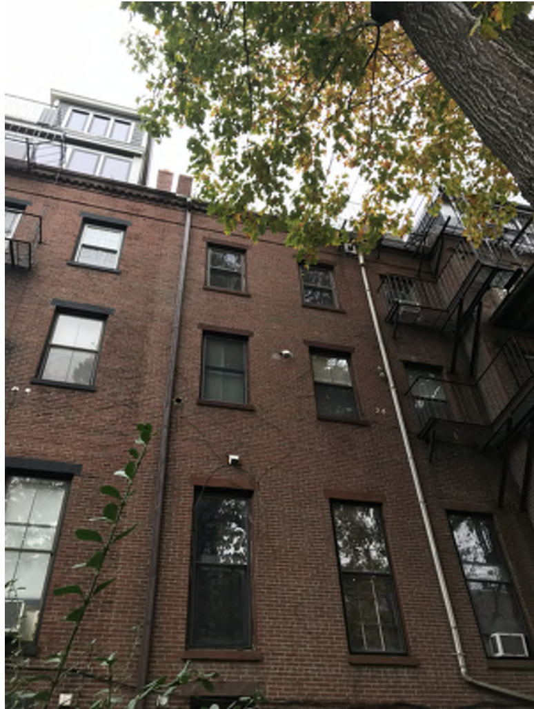
EXISTING REAR VIEW OF CHIMNEY
