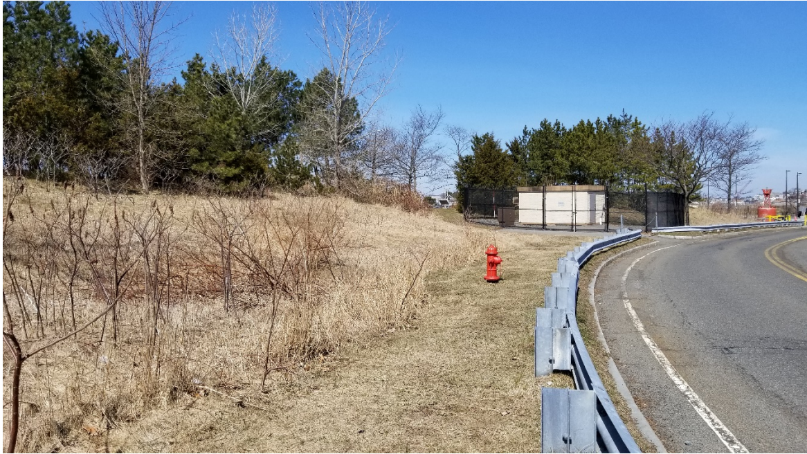
Photo 3. Proposed parking lot project area (looking northwest). The parking lot will accommodate nine parking spaces (two of which will be handicap accessible) and will provide public parking for the proposed public fishing pier (separate project) to be located to the west on Boston Harbor.
