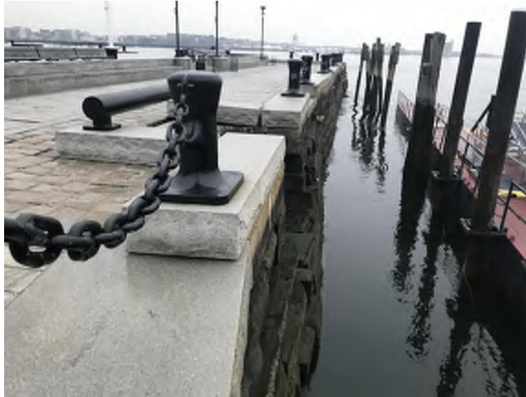
Existing Seawall Looking East from Topside
