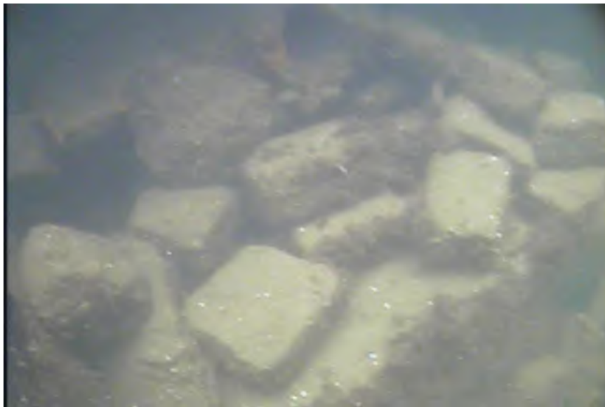
Typical Seawall Condition in Proposed Repair Area
