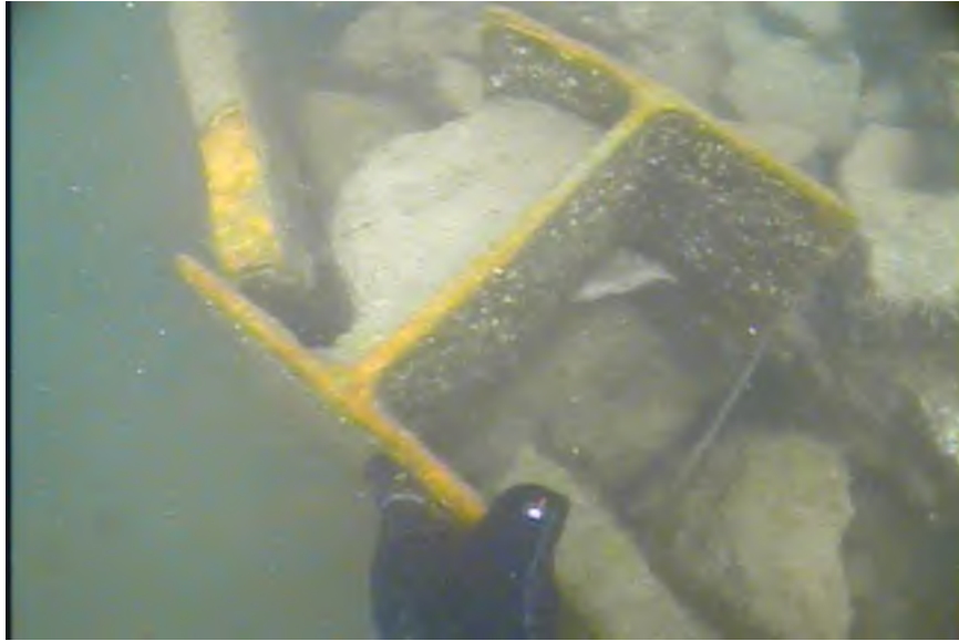
Previous Seawall Repairs from Dive Inspection
