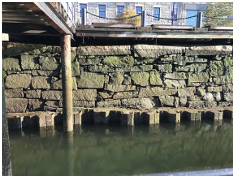
Previous Seawall Repairs Looking North from Floats
